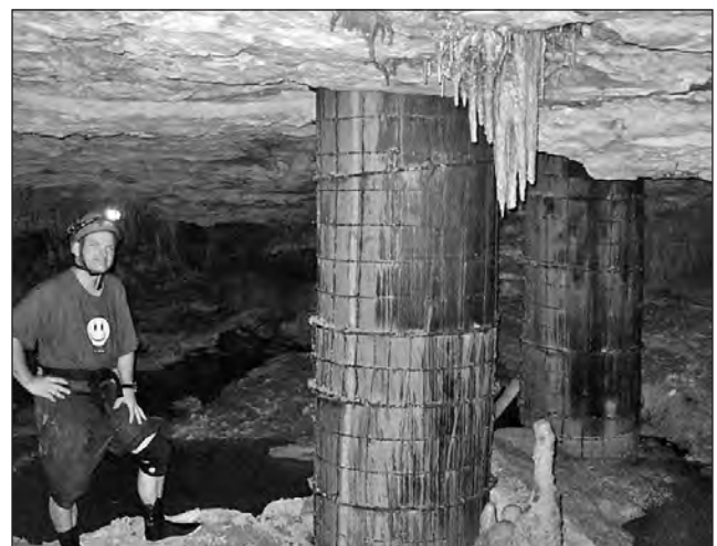
Support pillars for a pedestrian overpass extend into Cueva Aluxes. Left, Patricia Beddows; right, Pat Kambesis.
