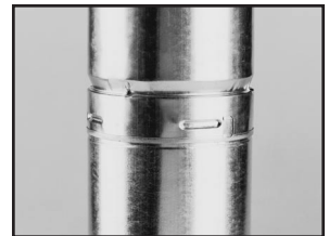
Push the ends of the pipe together.
