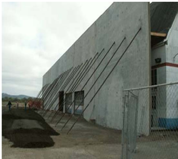
Source: Concord Construction Company
