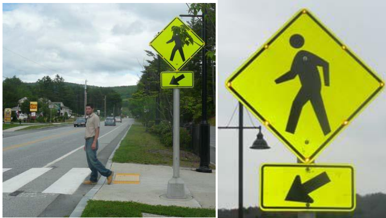
Figure 73: A pedestrian sign with blinking lights installed at a crosswalk.
