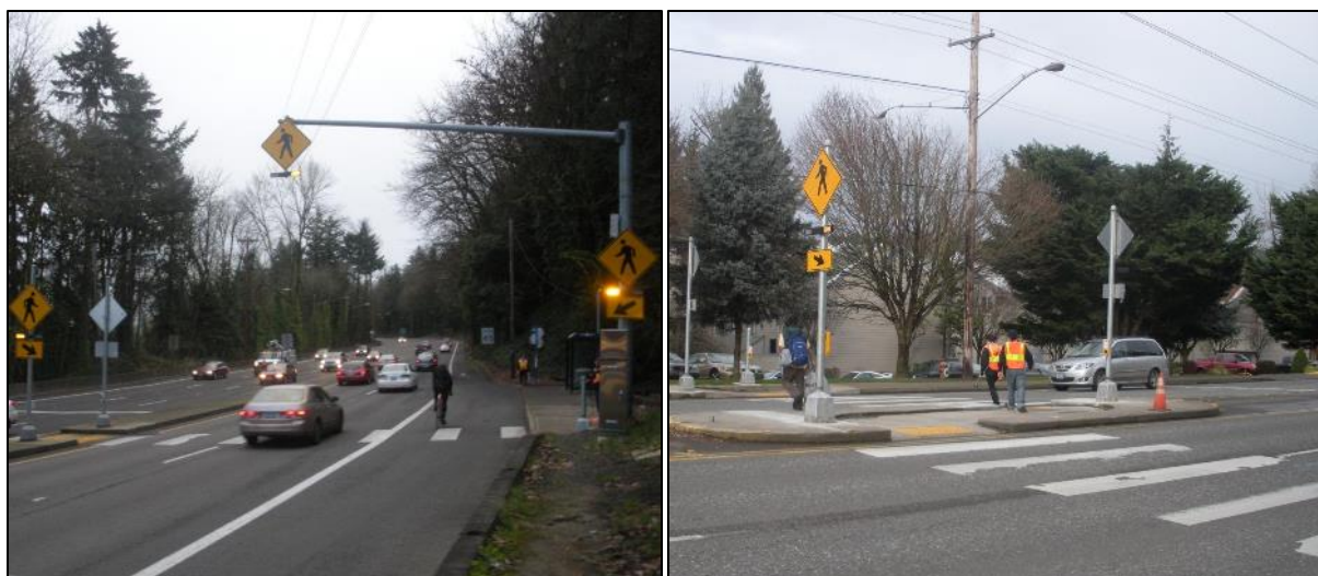
Figure 60. RRFB installation in Portland, Oregon
