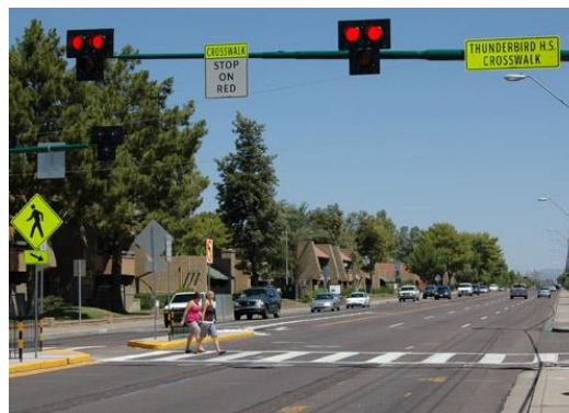
Figure 53: Pedestrians cross at a crosswalk enhanced with a pedestrian hybrid beacon in Phoenix, Arizona
