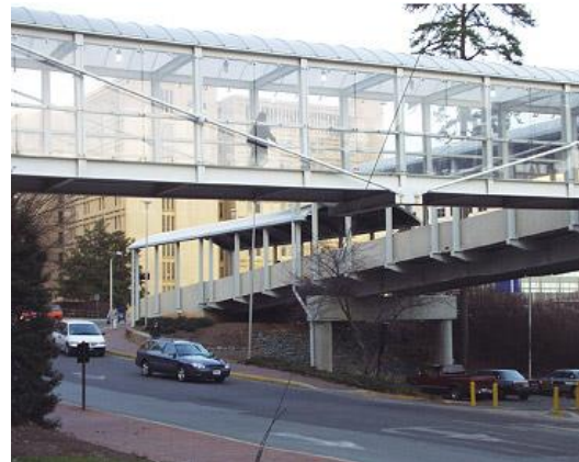
Figure 21: A pedestrian overpass.
