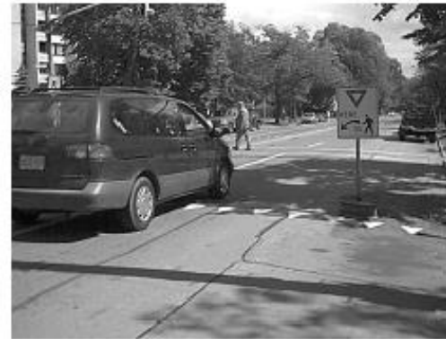
Figure 45: A pedestrian crosses while a vehicle waits at the advance yield markings.
