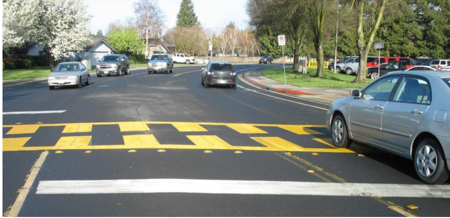
Figure 77: A high-visibility yellow crosswalk in Stockton, California
