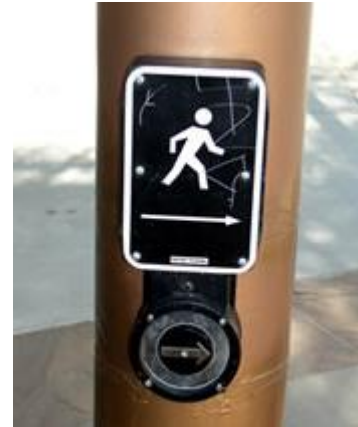
Figure 51: A pedestrian call button that provides audible and visible response when pressed
