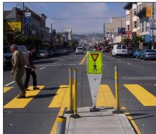
Figure 67: Two pedestrians use a high-visibility yellow crosswalk that has been enhanced with an in-street pedestrian sign in San Francisco, California.
