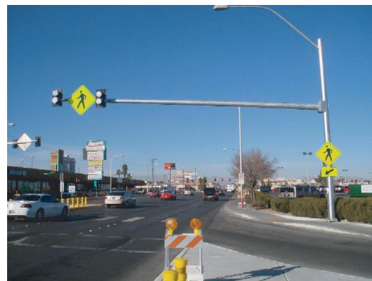
Figure 9: A pedestrian-activated flashing yellow signal.
