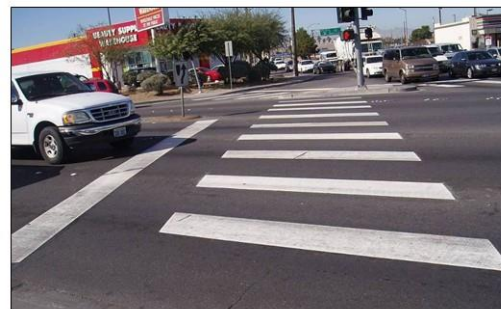
Figure 7: High visibility crosswalk at an intersection in Las Vegas.
