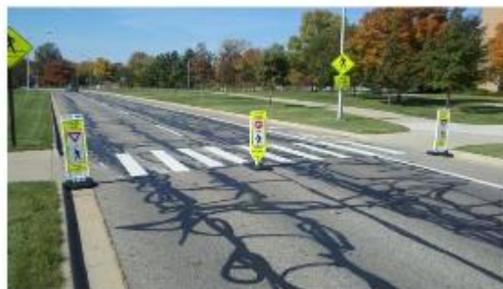
Figure 69. The gateway configuration of In-Street Yield to Pedestrian Signs
