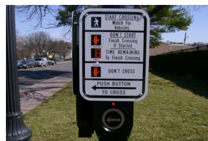
Figure 49: An accessible pedestrian signal, designed to provide cues for visually- and hearing-impaired pedestrians
