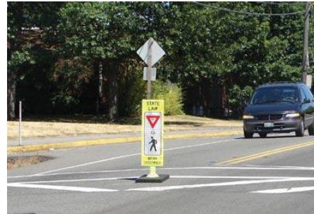
Figure 65: In-roadway pedestrian sign installed mid-crosswalk
