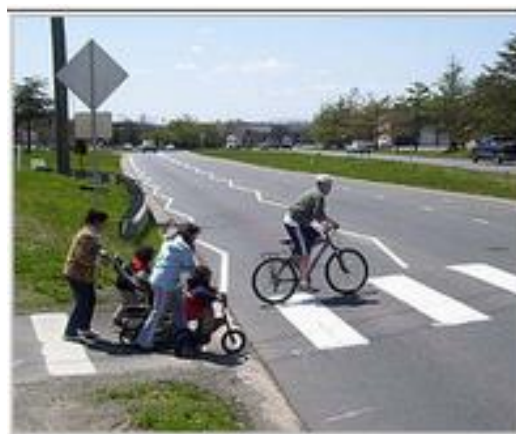
Figure 12: Zig-zag pavement markings used in Virginia to call attention to the presence of pedestrians.
