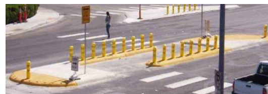
Figure 17: A Danish offset median refuge island as used in Las Vegas, Nevada.
