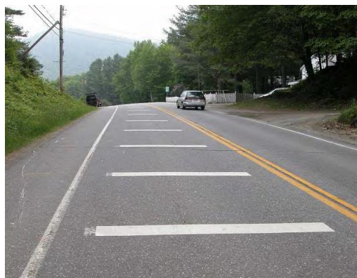
Figure 34: Dynamic Striping along Vermont Route 30.
