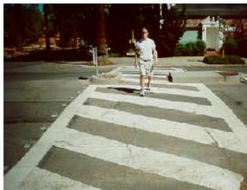
Figure 14: A pedestrian crosses in a zebra crosswalk that has been enhanced with a refuge island.
