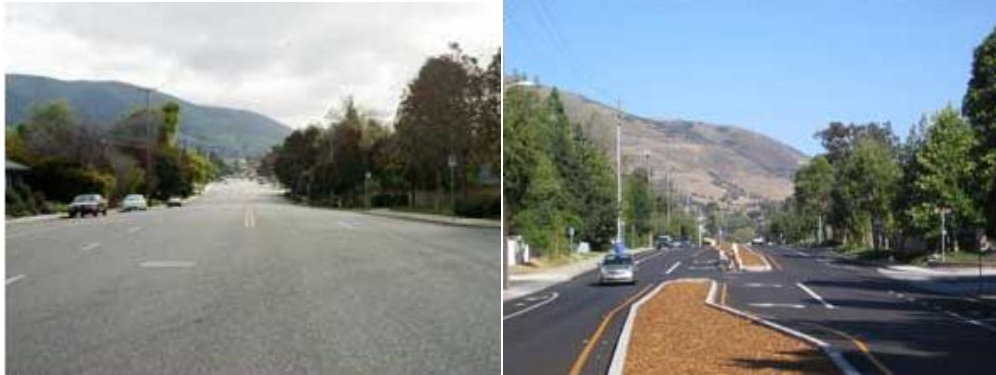
Figure 28: Before and after pictures of a road diet project in California.
