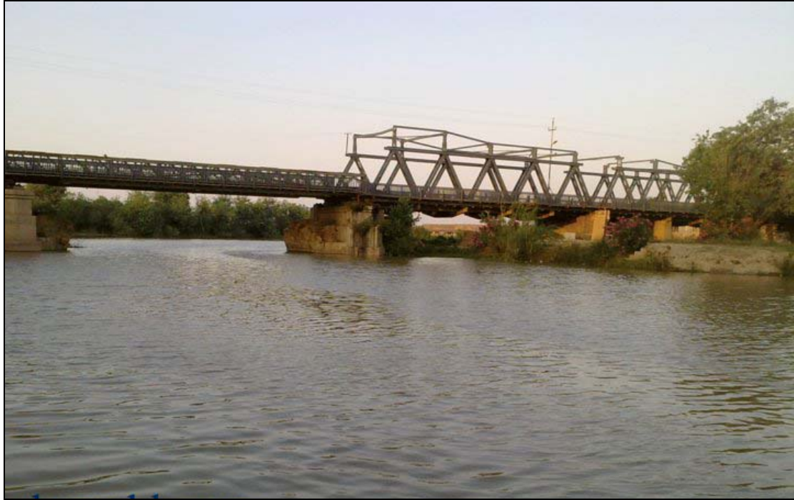
Figure (3) Altunköprü Bridge, photo by Ali Kassap
