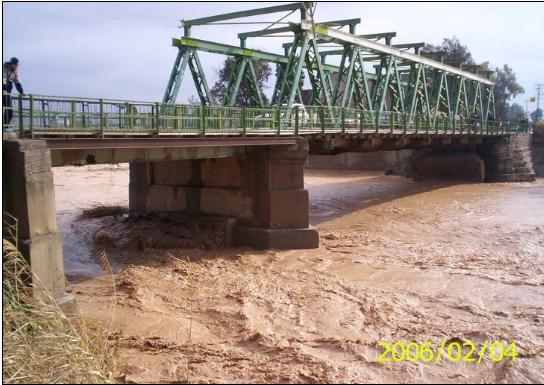
Figure (4) Altunköprü Bridge, photo by Ali Kassap
