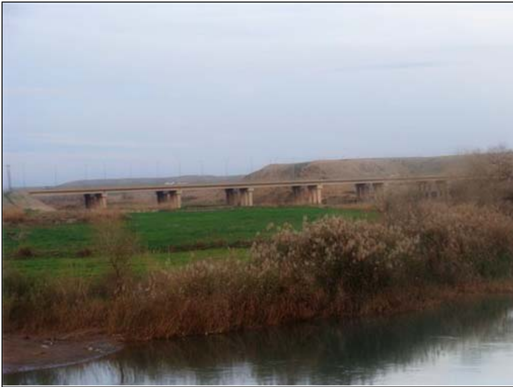
Figure (14) scenery from Altunköprü
