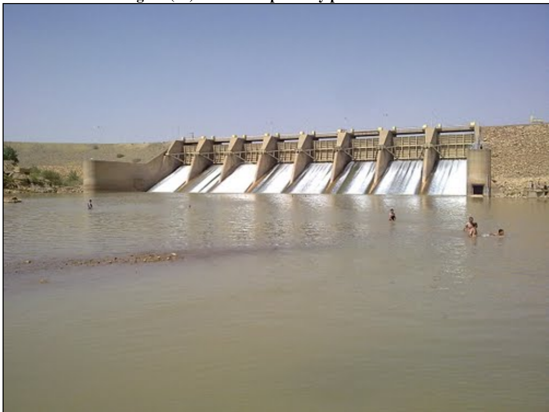
Figure (13) Dibilis Dam photo by panoramio.com. The dam is located directly north of the district of Dibilis (Numera Sekiz) in Kirkuk. The main-purpose of the Dibilis Dam is to divert water from the little Zab River into the Kirkuk Irrigation project.
