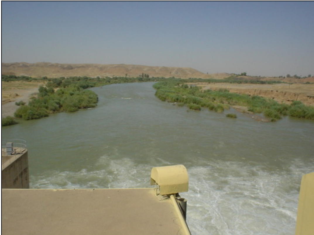
Figure (12) Dibilis Dam photo by panoramio.com
