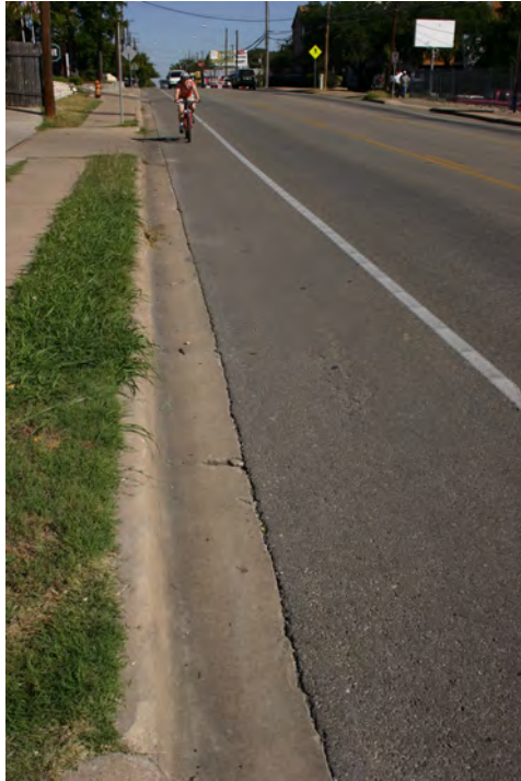
Figure 7.6. Example of a smooth seam between a gutter pan and roadway
