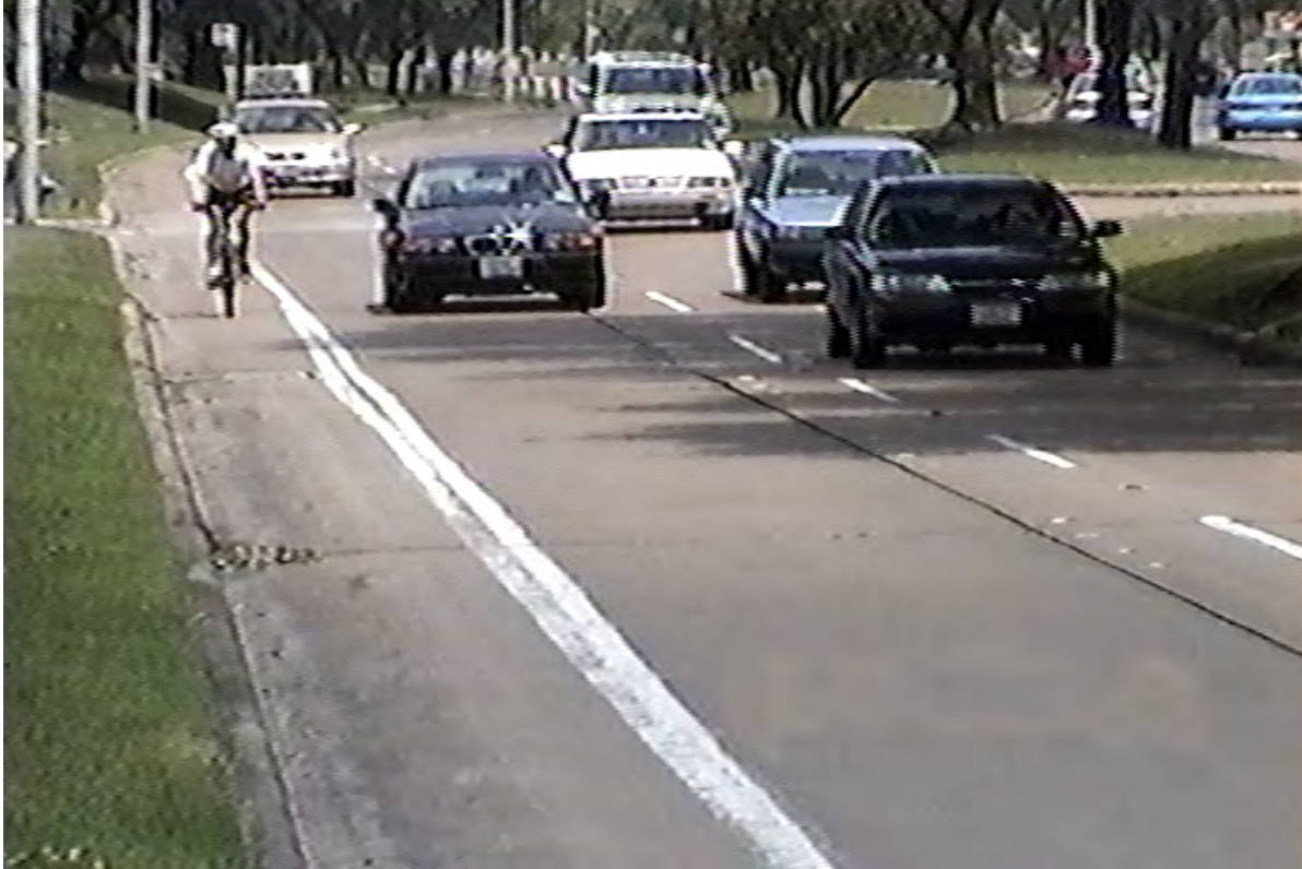
Figure 7.23. Typical cyclist and motorist lateral position on a roadway with a bicycle lane (10 ft motor vehicle lane and 4 ft bicycle lane)
