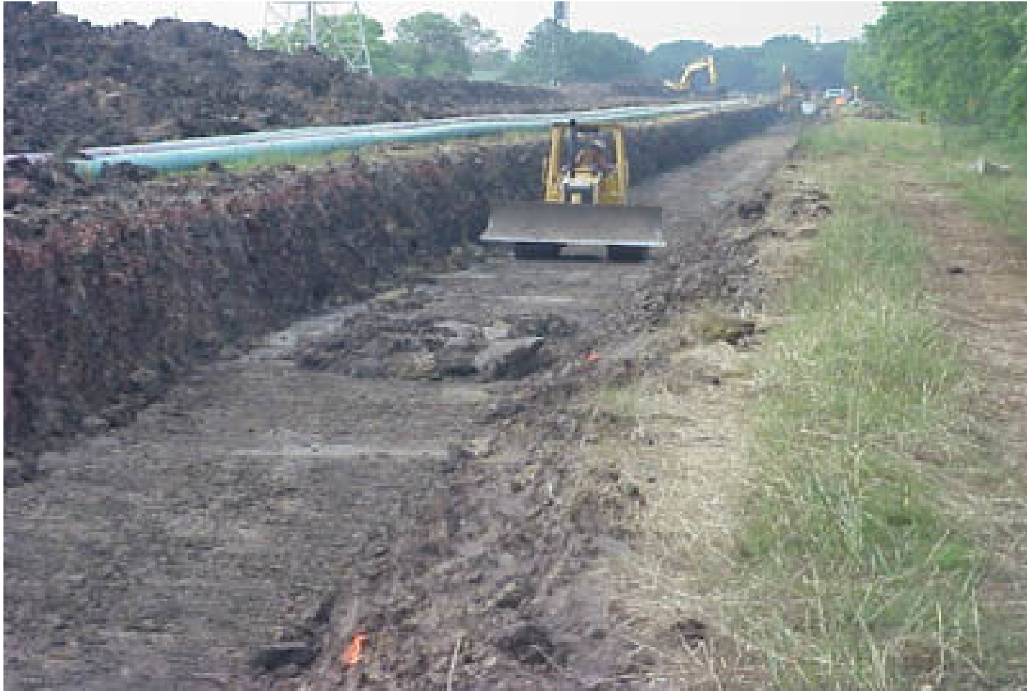
Multiple pipeline trench - Baytown, TX
