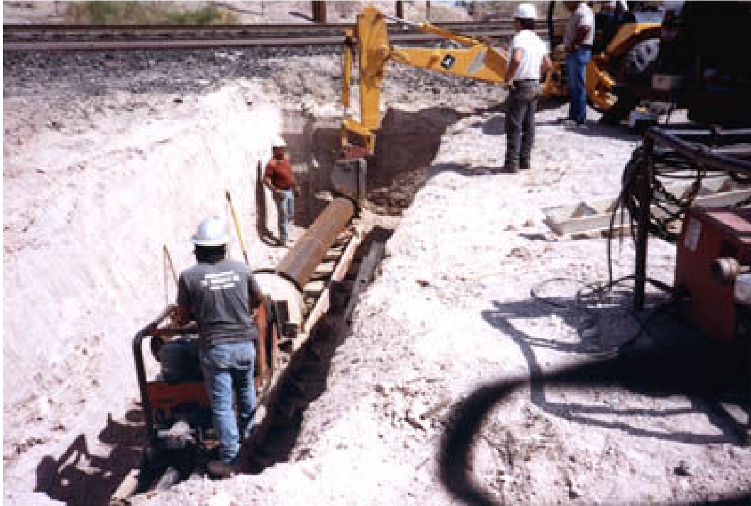
Horizontal bore of railroad
