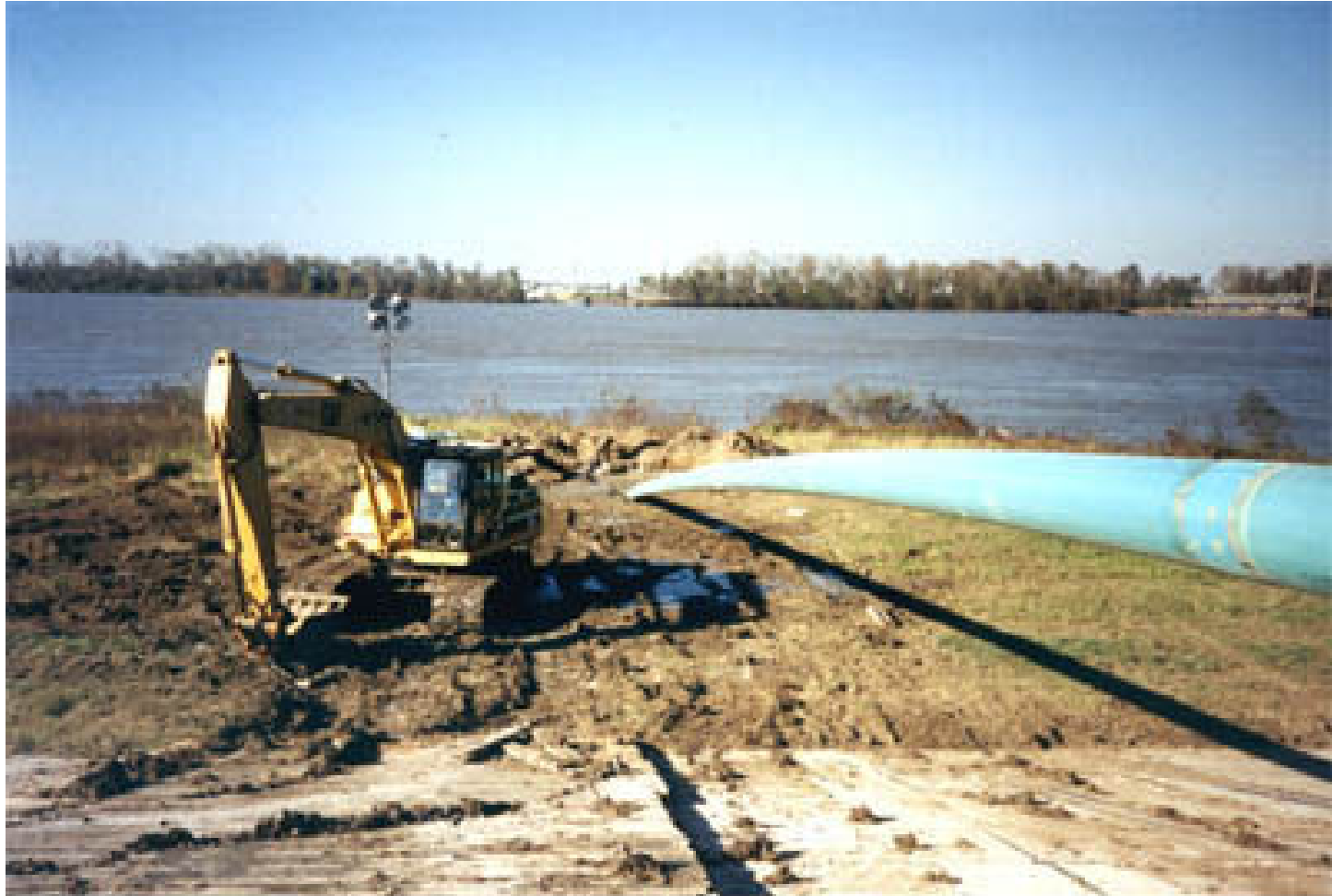
Hydrogen pipeline - Mississippi River Crossing
