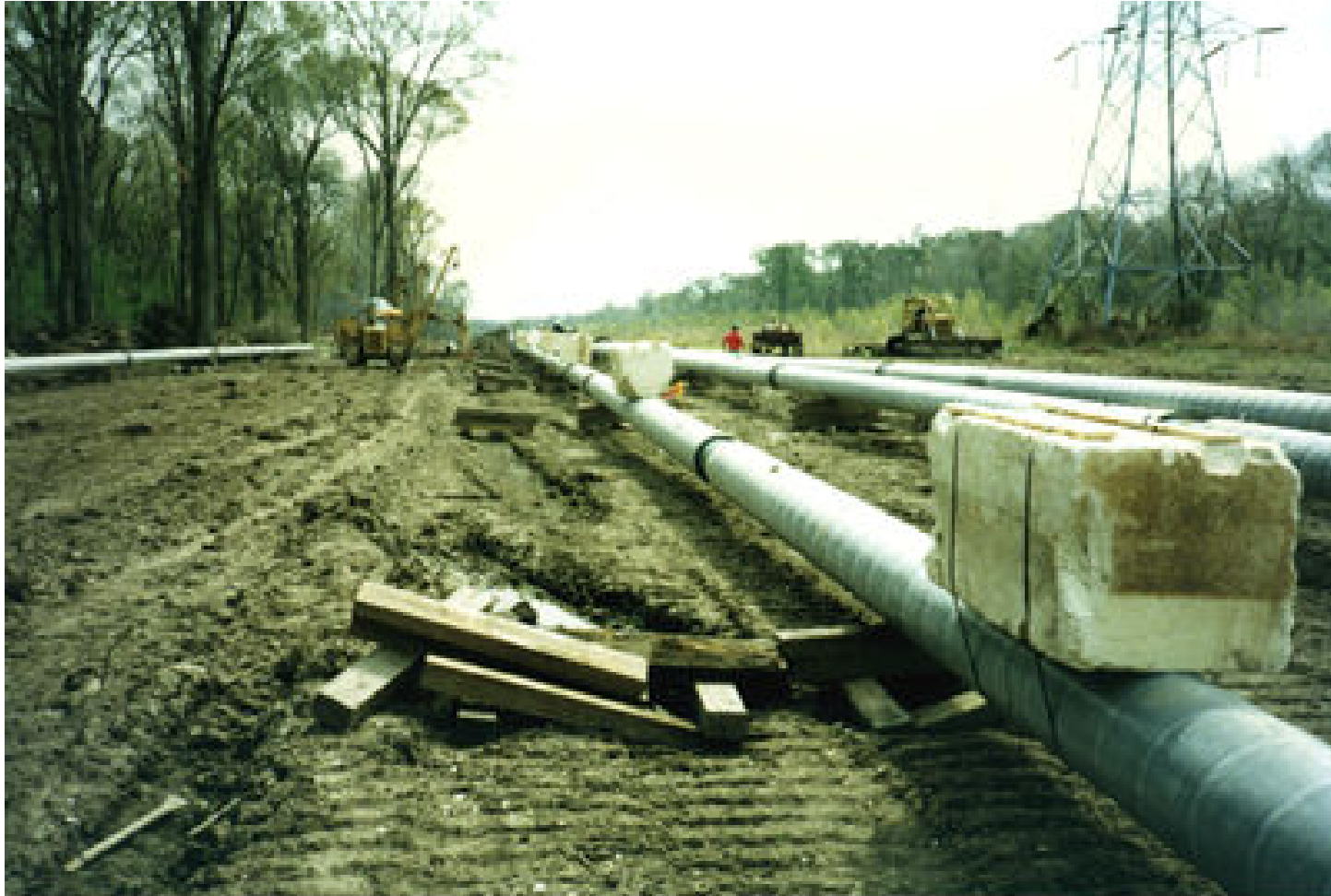
Concrete coated pipeline with floats in Taft, Louisiana
