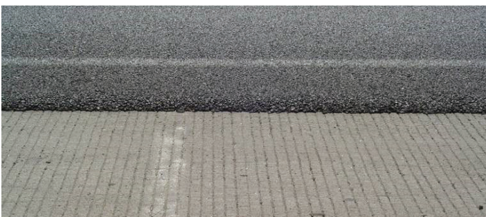
Figure 3. Quieter pavement overlaying louder pavement, Arizona Quiet Pavement Pilot Program. From Donovan et al., 2012.
