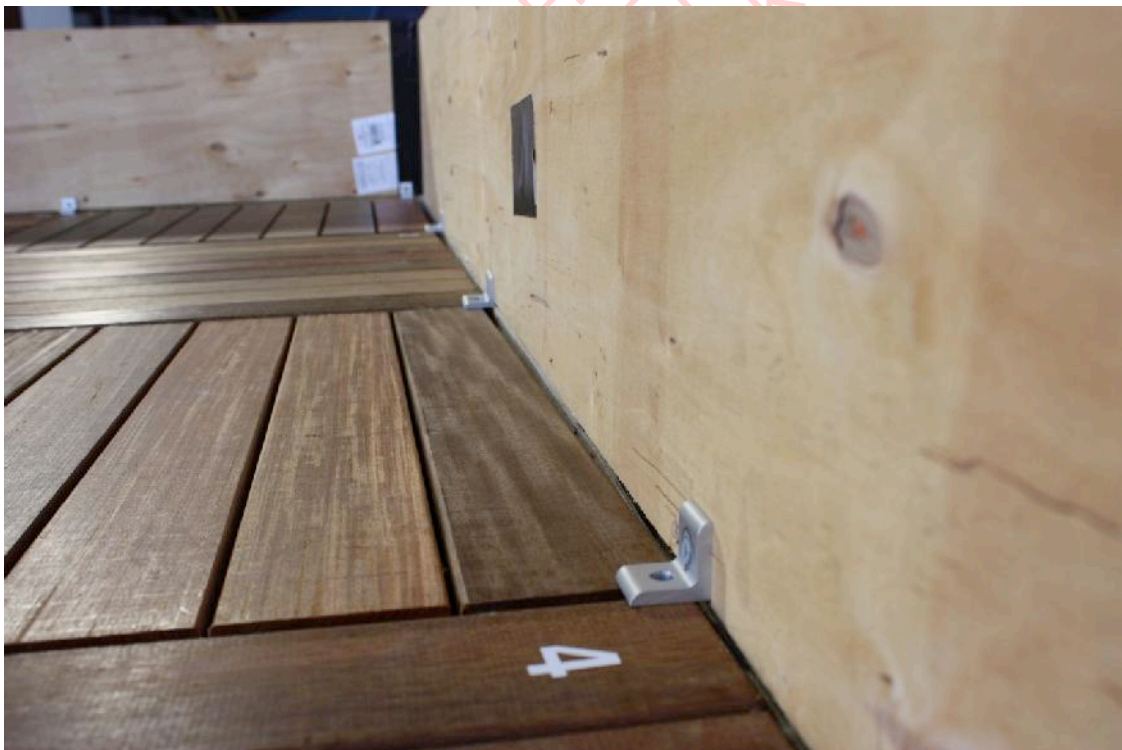
Figure 11 - Detail of the perimeter paver locking devices
