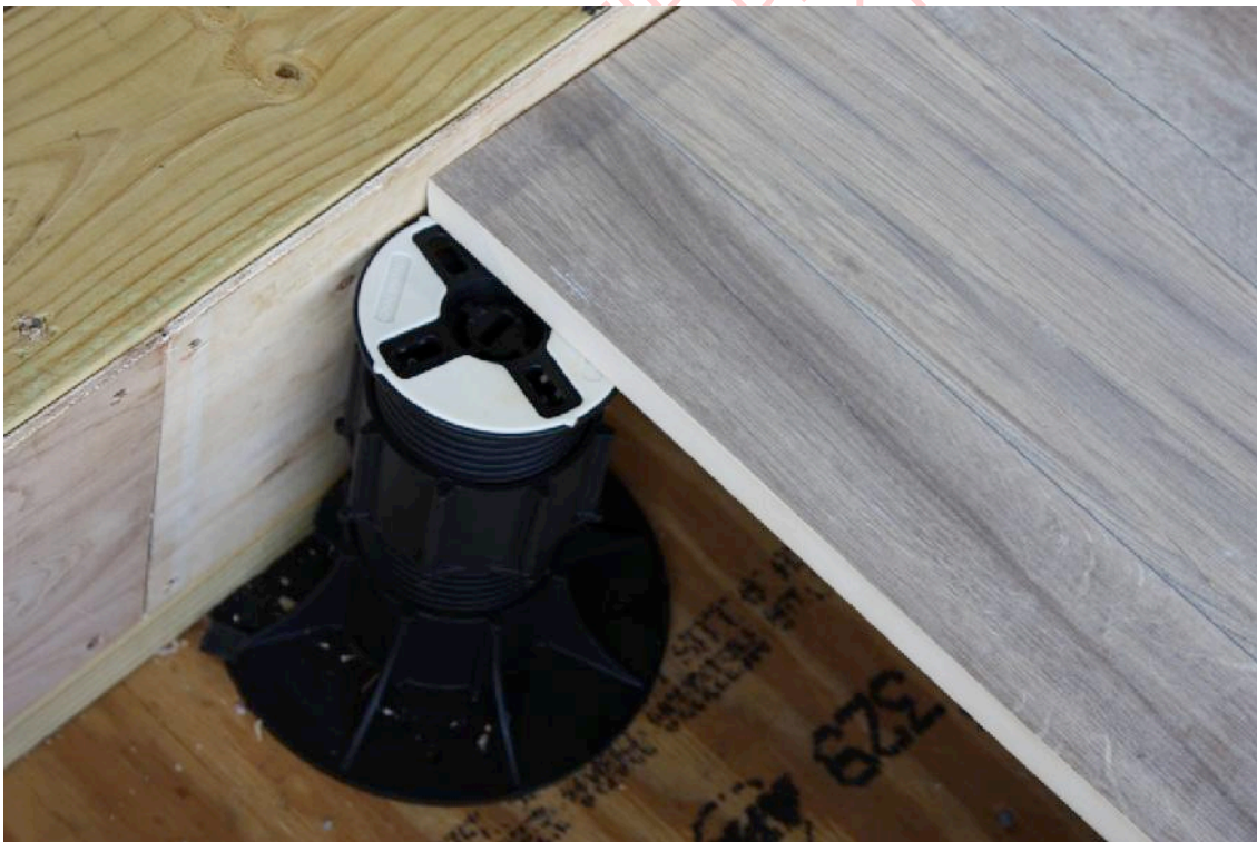
Figure 13 - Close up of a perimeter pedestal. Some rotation of the pedestal cap plate can be seen.
