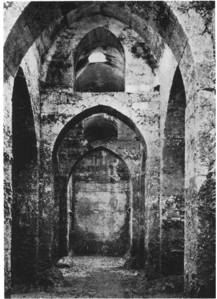
b. RAMLA. Cistern, entirely built with pointed arches and dated 172/789.
