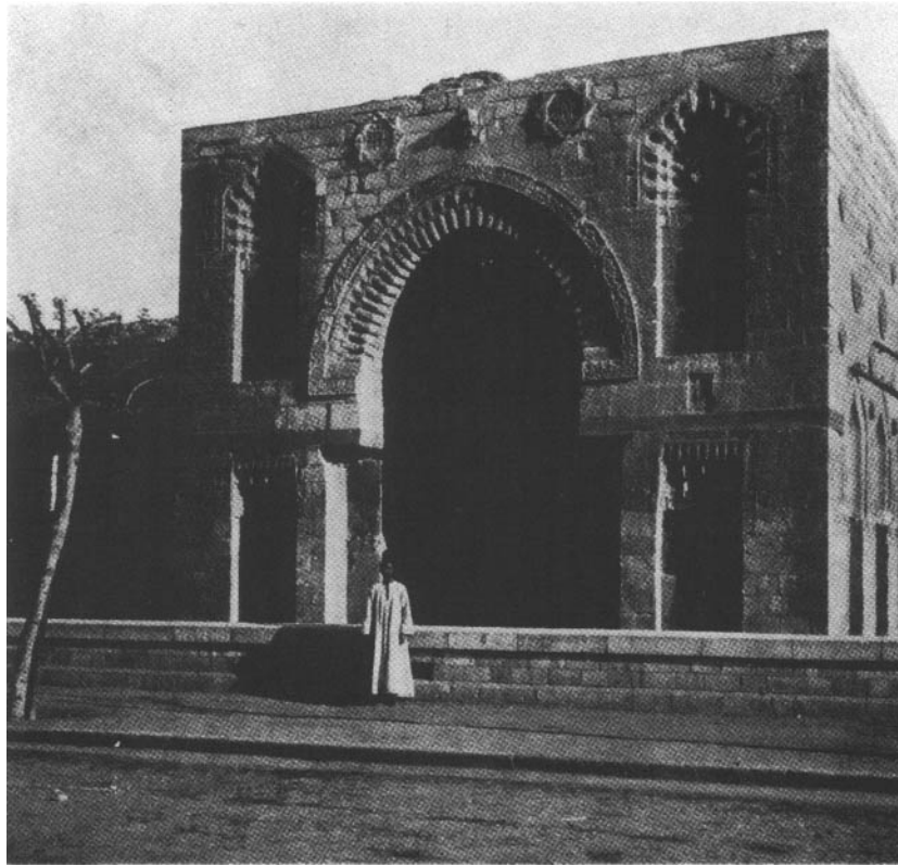
b. CAIRO: Mosque of Baybars, north-western entrance. 665/1267.
