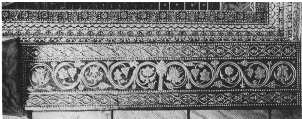
c. THE DOME OF THE ROCK. Bronze covering on under-side of tie-beams.
