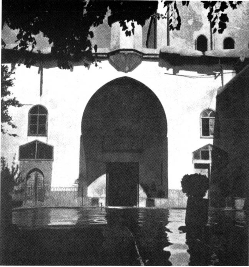
5. Courtyard of the Madrasa al-Nūriyya, interior of the eastern façade By courtesy of the General Directorate of Antiquities, Damascus
