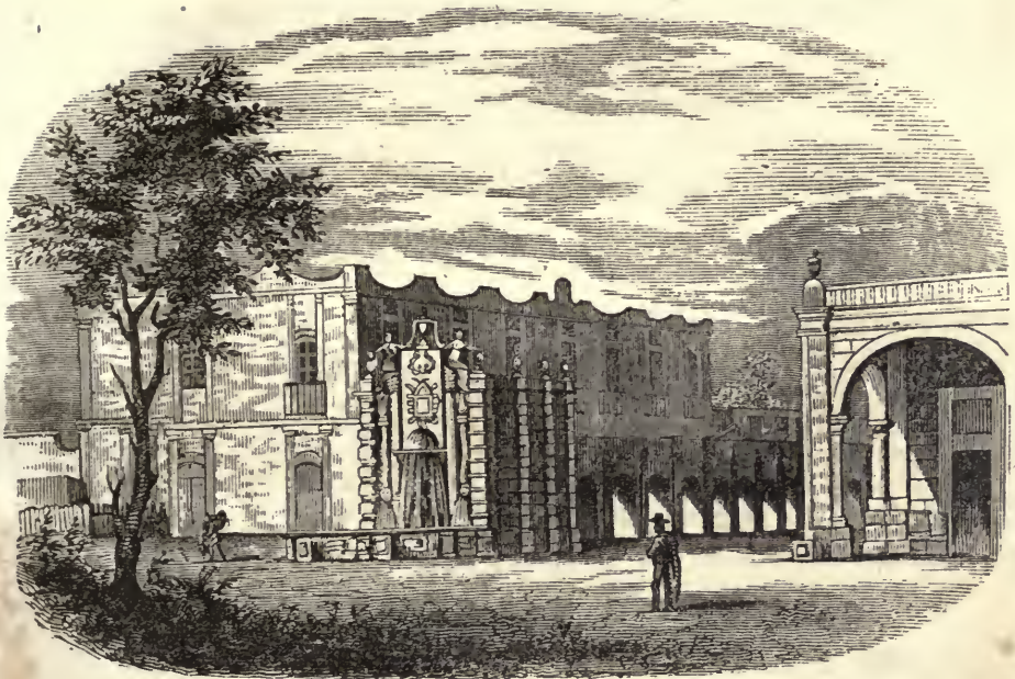
Termination of the Aqueduct in the City of Mexico.
