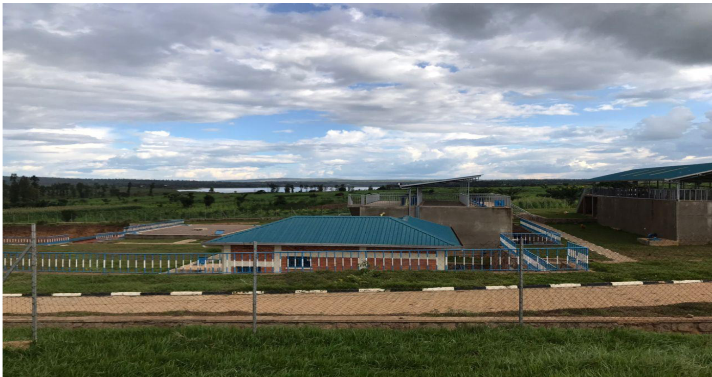
Figure 4: WASAC water intake facility near Gashora wetlands
