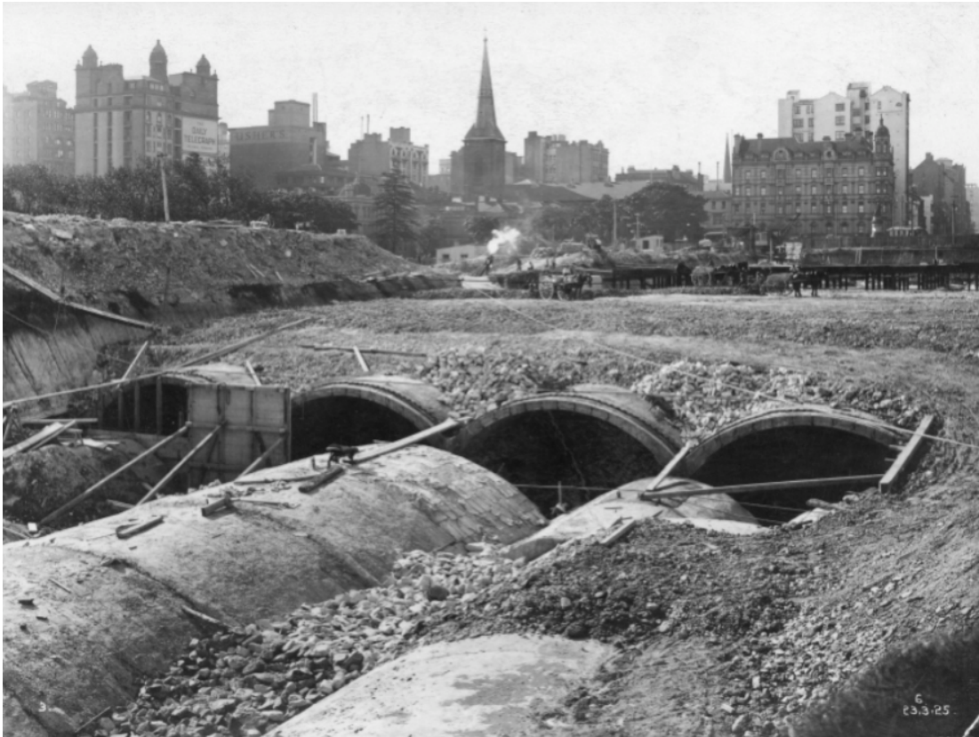
Starting to recover St James Station. Note how close it is to the surface.
