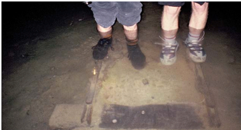
Construction railway under Lake St James.
