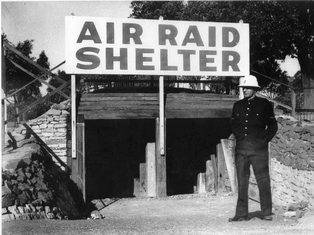
The entrance to the air raid shelter in Hyde Park South.
