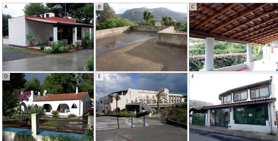
Fig. 6 Typical buildings on the island of Vulcano. A–C Most representative type of residential building, typically single-storey with a concrete flat roof ( B ) and a timber front porch ( C ). D residential building with a roof made of a timber structure and tiles. E Typical one to three storeys hotel complex and F typical commercial arcade in the Porto area. Following the classification of (Spence et al, 2005), buildings shown in A, B, C and E are classified as medium strong (MS) or strong (ST), and buildings D and E as weak (WE) or medium weak (MW).
