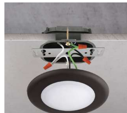
J-BOX MOUNT INSTALLATION (for 4" housings)
