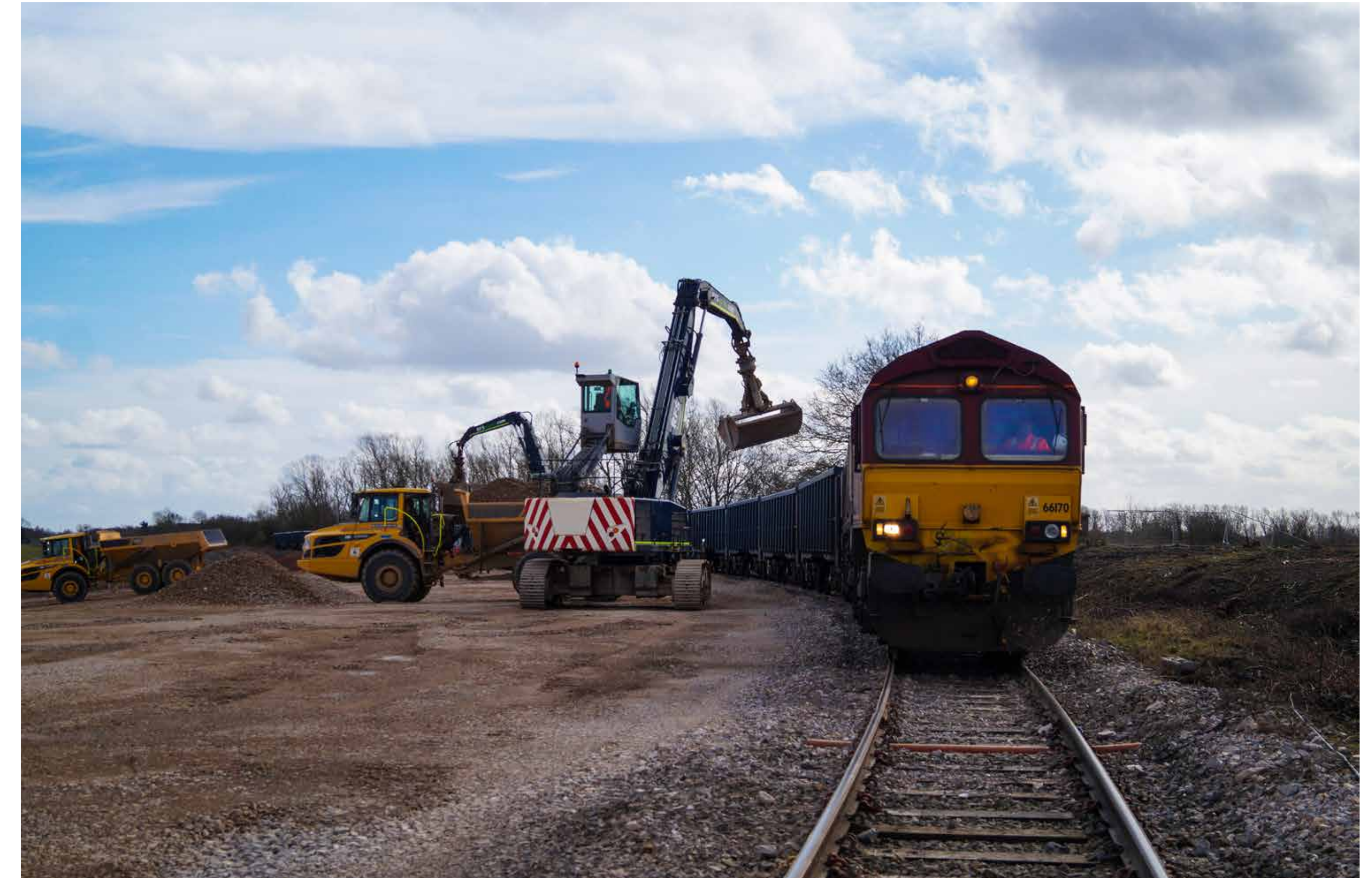
Freight trains delivering construction material
