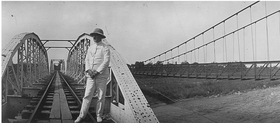
A railway and a pedestrian bridge, East Java. (KITLV)
