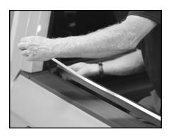
C. With side rail guide set on top of box, position side rail tight to front of box. Working from front of box to rear, adhere side rail to inside edge of box rail.
