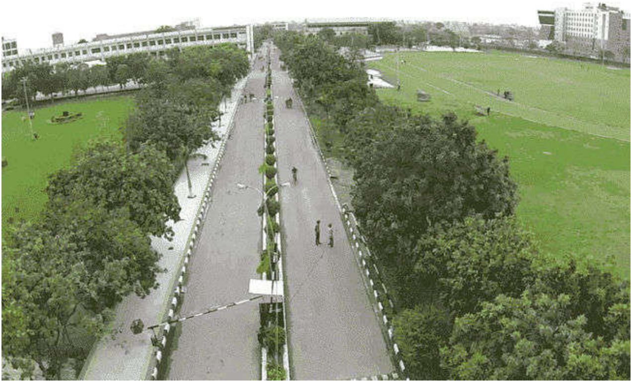
Photo 4: Main Entry Road of College Campus
