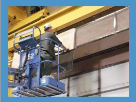
Coleman Tool's welding smoke is eliminated by air curtains outfitted with quickaccess, MERV 8 air filters designed by maintenance staff.
