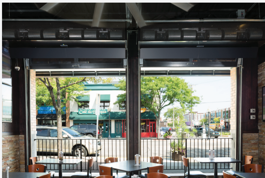
Berner Industrial Direct Drive 12 Air Curtains over the open wall
