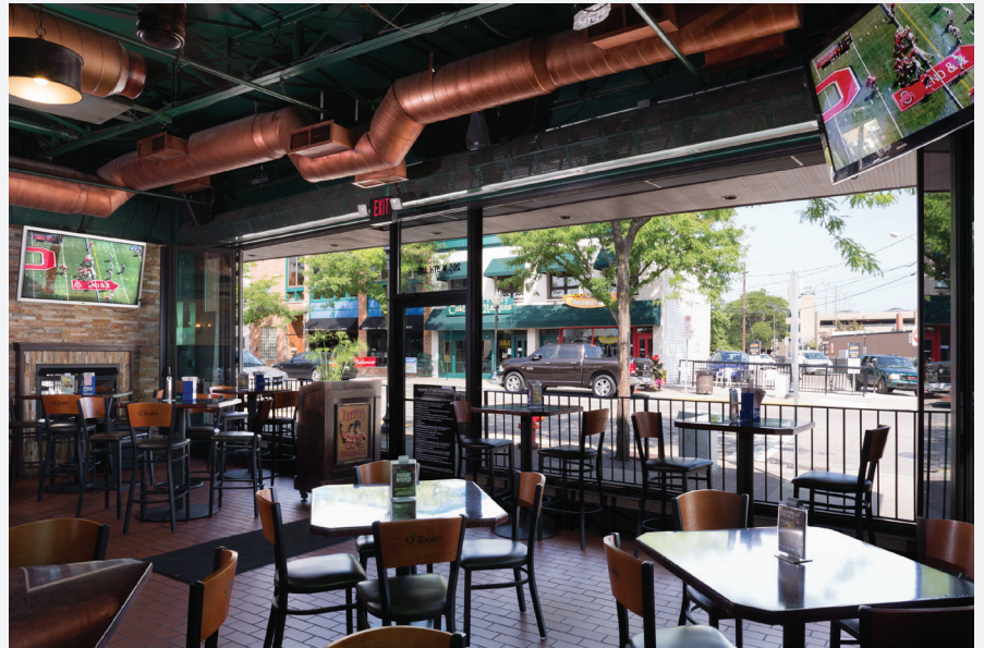
Berner Commercial High Performance 10 Air Curtains over the open wall
