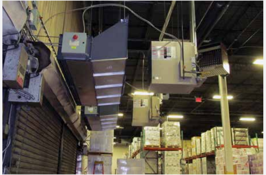
Berner Industrial Direct Drive 12 with indirect gas heat Air Curtain over Shipping Door
