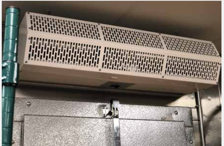
Berner Commercial Low Profile 8 Air Curtain over a Walk-in Cooler
