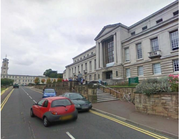
The Portland and Trent Buildings
