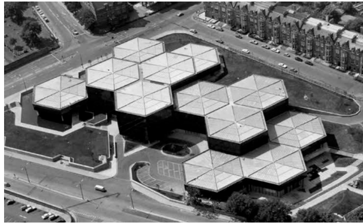
Above: Plan consists of 12 linked hexagons beneath Salisbury Crags, opposite: Glazed curtain walls feature manganese bronze mullions
