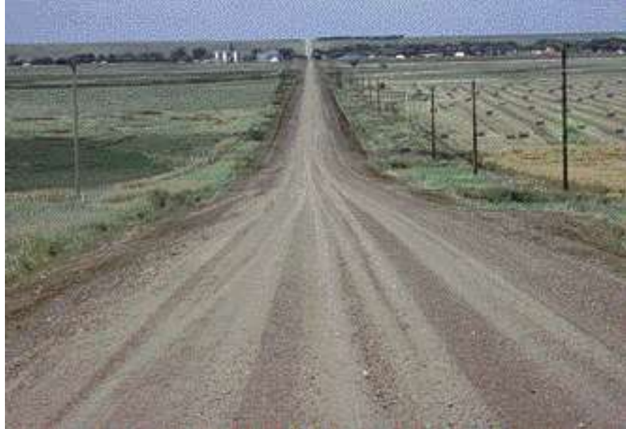
Example of a gravel road with good shape of cross section. Notice crown in driving surface and proper shape of shoulder and ditch.
