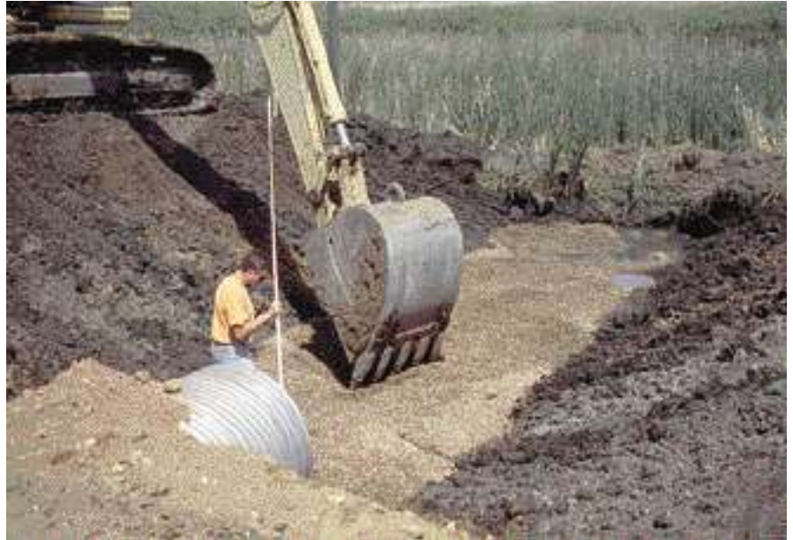
New culverts installed well and at correct elevation are essential for carrying water under a road. A reasonable maintenance schedule is required to keep them functioning well.
