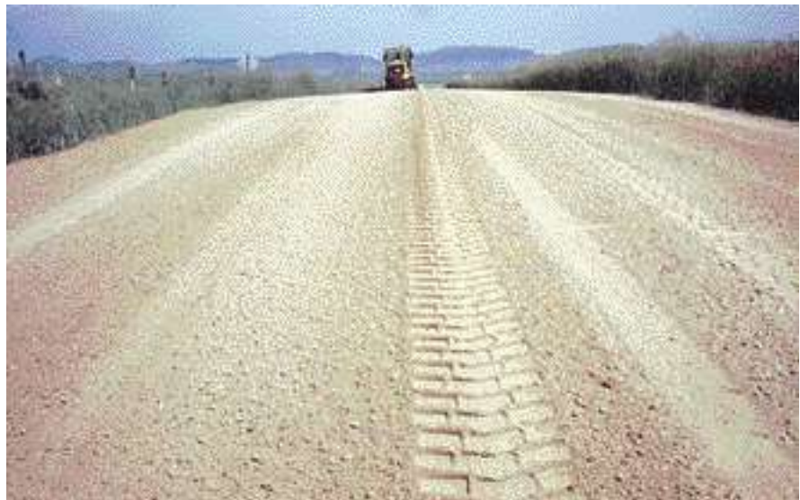
The carbide-tipped bits on a cutting edge can be a valuable tool in preparing a road for Chloride treatment. They penetrate the road and give a shallow scarifying effect to loosen and mix the existing gravel. This leaves a nice uniform loose layer of material on the surface.
