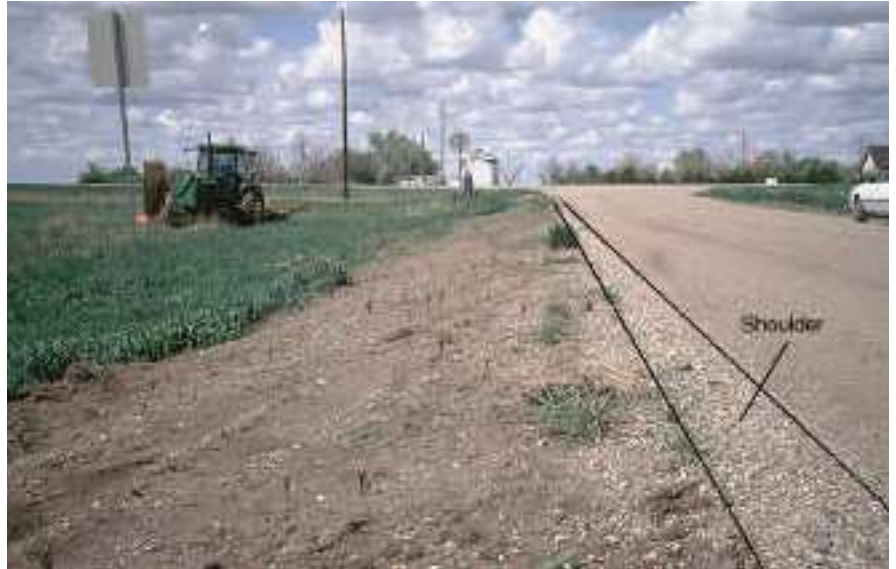
The photos above and below show good examples of gravel shoulders that match the edge of the roadway very well and drain water to the ditch.
