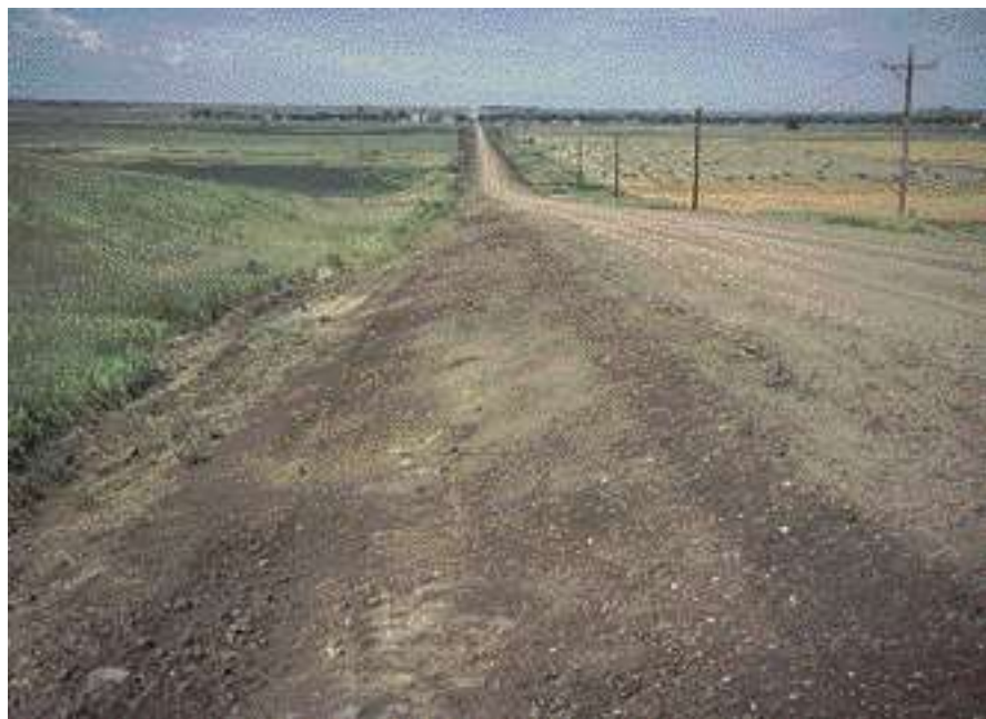
An example of a well shaped gravel road shoulder that slopes away from the driving surface and drains water to the inslope and ditch.
