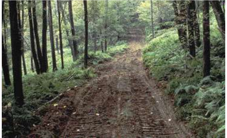
This gravel road with narrow right-of-way has turned to mud during wet spring conditions. It represents low-volume roads commonly found in several parts of the world.
