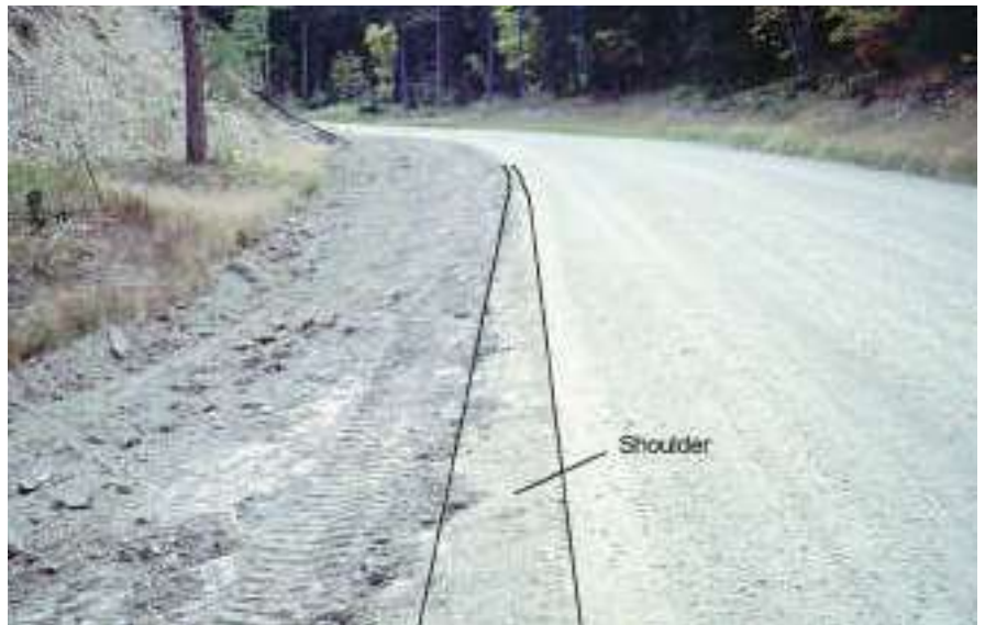
The photos above and below show good examples of gravel shoulders that match the edge of the roadway very well and drain water to the ditch.
