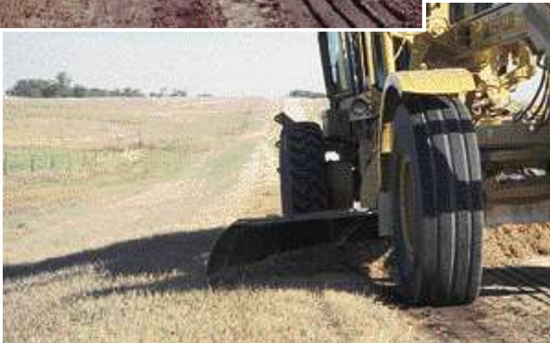
The material from the high shoulder is then pulled into the cut that has just been made. Generally, this material will have to be worked several times with the grader to break it up enough to spread evenly.
