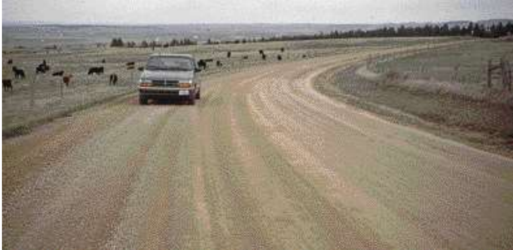
This superelevated road section makes driving safer.
