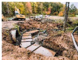
McConnell Contracting, Inc. from West Lafayette, Ohio constructs a reinforced concrete box culvert bridge on Plymouth Rd., T.R. 374 in Perry Township.
