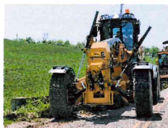
County bridge crew installing an in-house designed and fabricated flow improvement device to a bridge on Aster Rd., C.R. 17 in Perry Township (left); County forces berming Bear Rd., C.R. 28 in Loudon Twp. to improve drainage (center and right).
