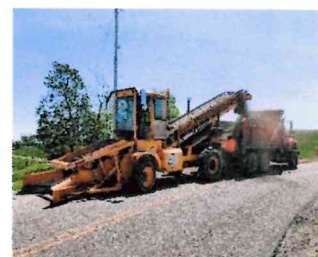
County bridge crew installing an in-house designed and fabricated flow improvement device to a bridge on Aster Rd., C.R. 17 in Perry Township (left); County forces berming Bear Rd., C.R. 28 in Loudon Twp. to improve drainage (center and right).
