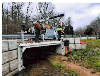
County bridge crew installing an in-house designed and fabricated flow improvement device to a bridge on Aster Rd., C.R. 17 in Perry Township (left); County forces berming Bear Rd., C.R. 28 in Loudon Twp. to improve drainage (center and right).
