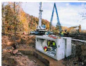
McConnell Contracting, Inc. from West Lafayette, Ohio constructs a reinforced concrete box culvert bridge on Plymouth Rd., T.R. 374 in Perry Township.
