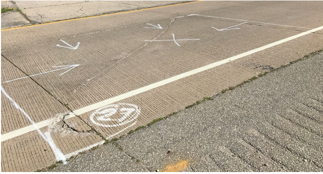
Figure 14. Clearly marked full-depth repair boundaries
