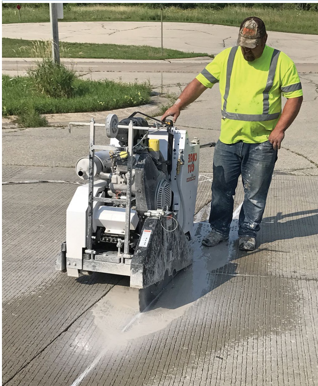
CP Tech Center (top) and Gerald Voigt, Square One Pavement Consulting LLC, used with permission (bottom)
