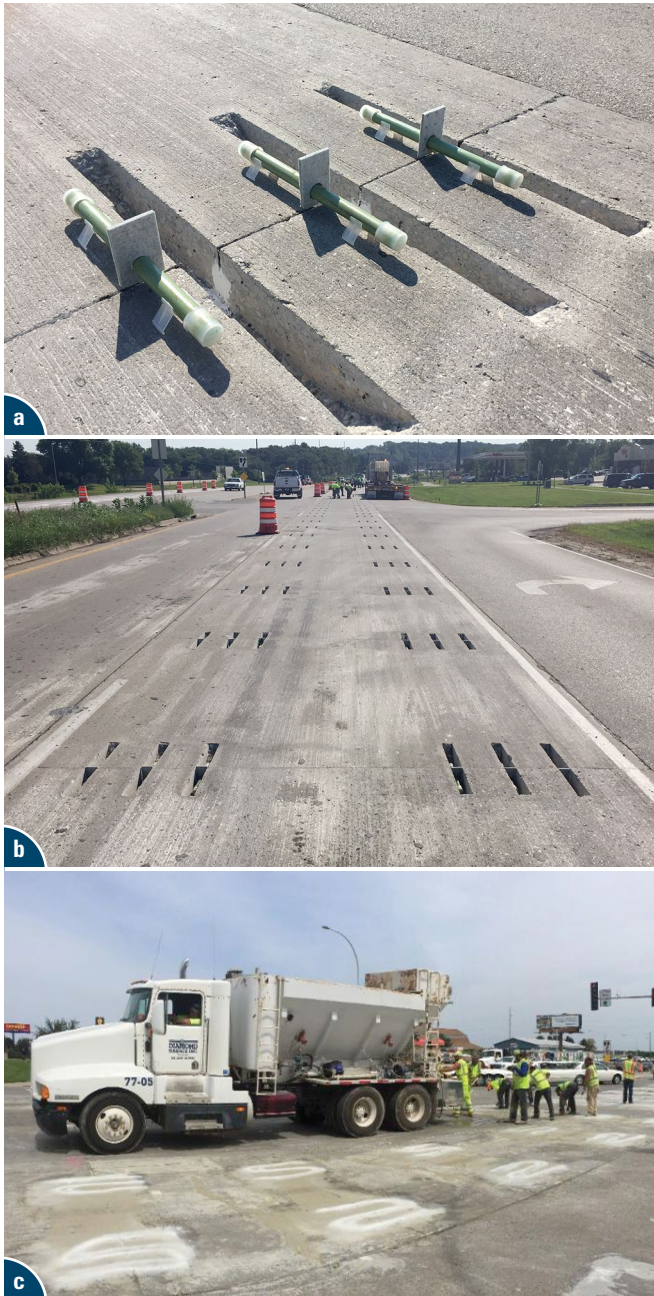
Figure 19. Dowel bar retrofit in a COA-U overlay in Olmsted County, Minnesota: (a) 1 in. bars, (b) bars inserted into parallel slots, and (c) backfilling
