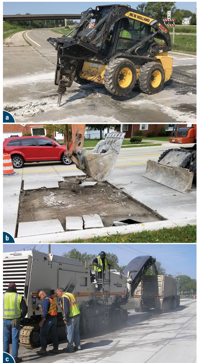
Figure 15. Removal methods for full-depth repair: (a) break-up and clean out, (b) lift-out, and (c) milling
