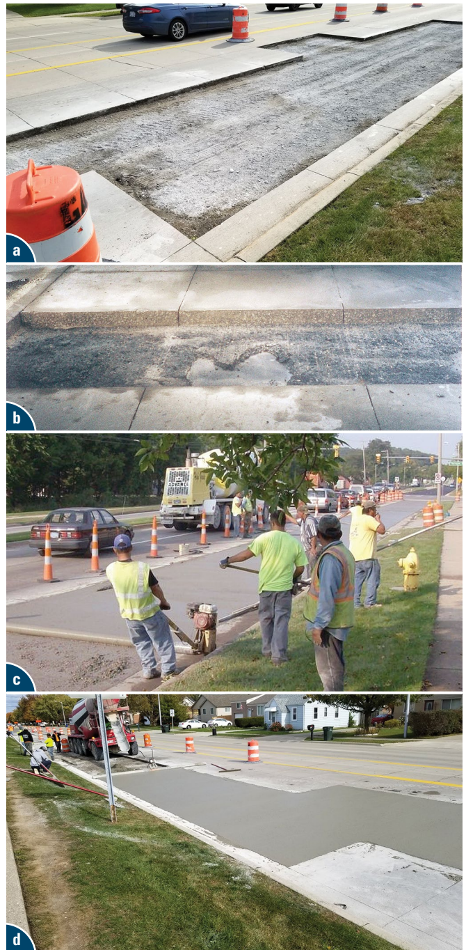
Figure 17. Placing and finishing a full-depth overlay repair: (a) COA-B removal area following joint lines, (b) COC-U removal area leaving the interlayer in place (note where a portion of the interlayer dislodged with the concrete), (c) screeding concrete in the repair area, and (d) concrete after screeding
