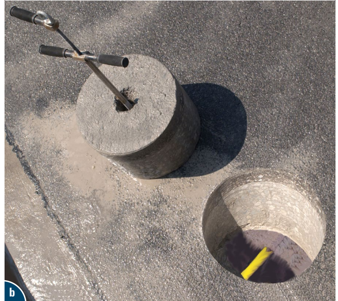
Figure 39. Keyhole coring: (a) truck-mounted keyhole coring drill and (b) example of a keyhole core removed from a pavement with an exposed utility pipe
