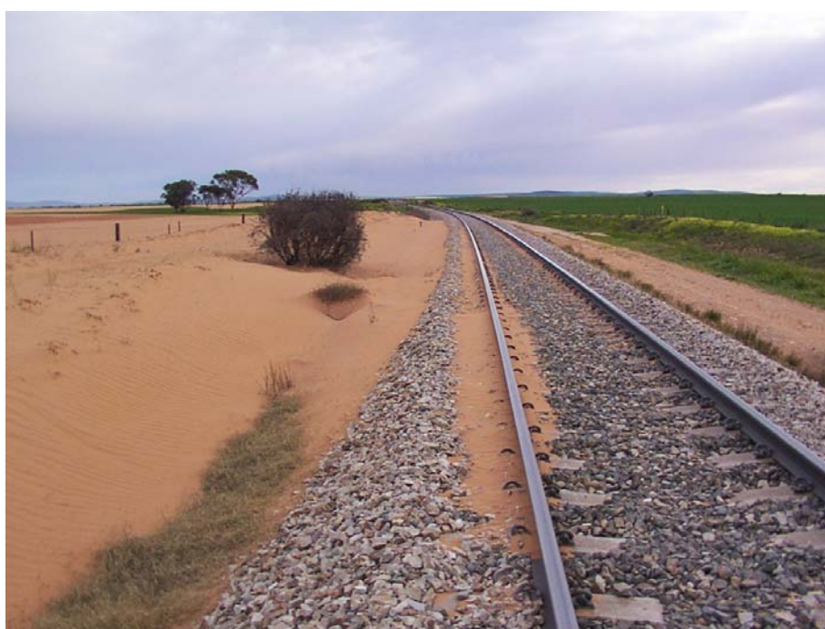
Figure 3: Moderate to High susceptibility to wind erosion land drifting in the NY region
