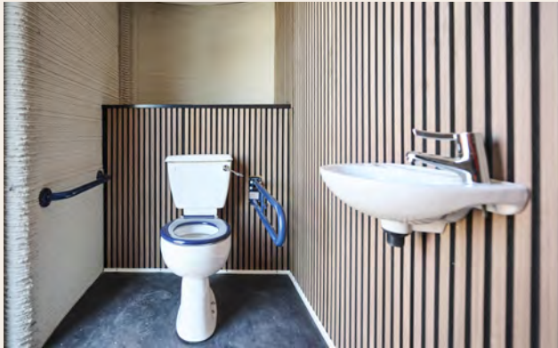
Inside the 3D printed toilet pod
