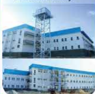
Construction of GYB Model Science Secondary School, Adankolo Lokoja
