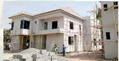
Ongoing renovation of Governor's Lodge, Abuja
