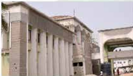
Ongoing renovation at the Taraba State House of Assembly Complex
