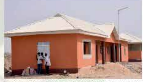
Jalingo modern Abattoir, at different stages of completion
