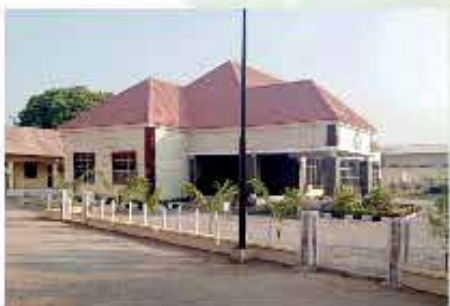
The newly renovated SSG's office
