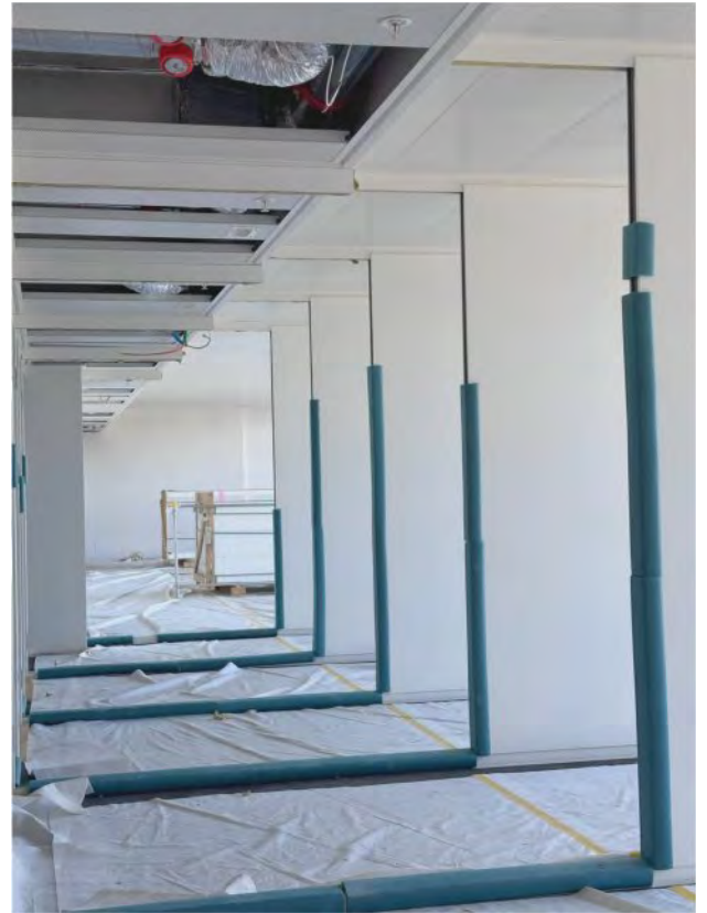
7 th floor: With some of the office partitioning partially installed.
