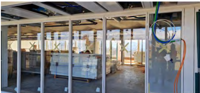
7 th floor: In line with the B building, small meeting rooms are being installed, and like the offices, they will have glass fronts and doors to increase the amount of natural light in the corridors.
