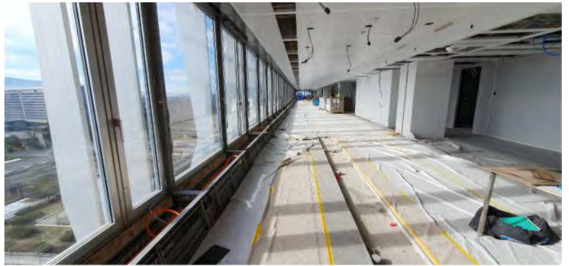
7 th floor: Before the office partitioning is installed.
