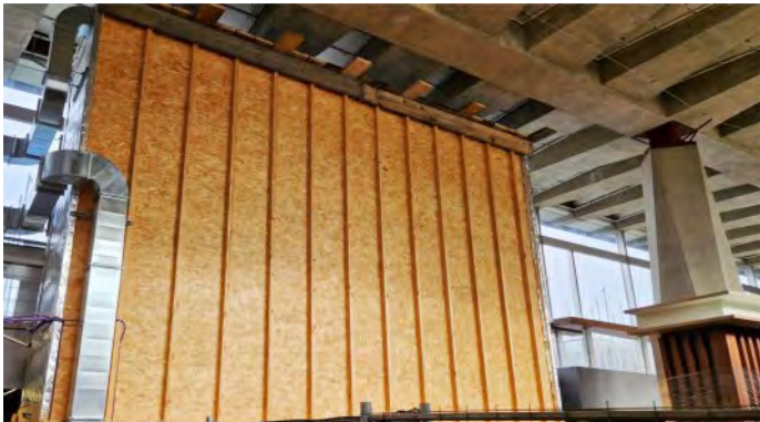
Basement level 1: This is the "Brazil" painting in its protective casing, with full temperature and humidity control.
