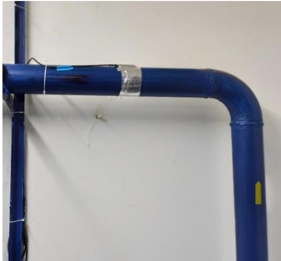
Figure 12. Sensor mounting.
