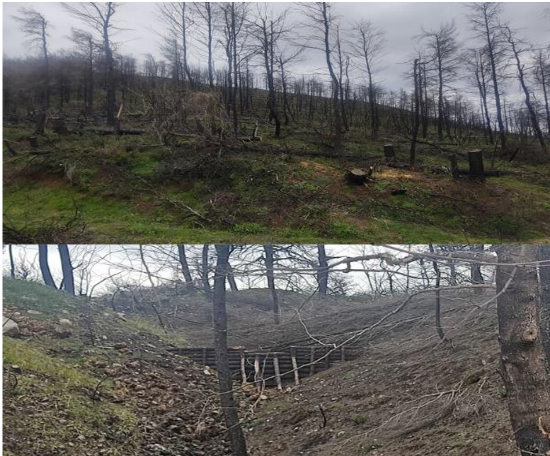
Figure 3: Soil protection and flood prevention structures in Limni. (Source: author's personal archive)
