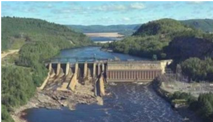
La Tuque dam and hydroelectric generating plant (date unknown) (photo source Hydro-Québec website)
