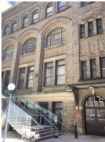
Basement entrance of the Electrical Building (Roseburgh Building). Legget's soil mechanics laboratory was in this basement. The staircase to the left leads to the Donnelly Centre opened in 2005. (photo Doug VanDine 2019)
