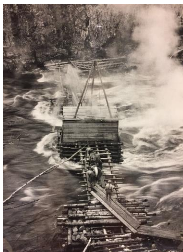
Photo of drill set up on Montreal River (photo by Legget)
