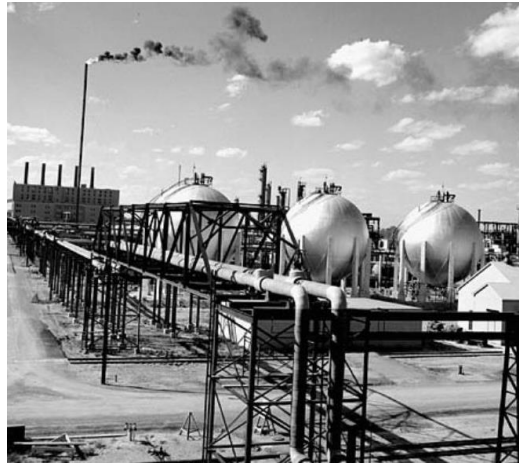
Sarnia Polymer plant, 1944, (photo source LAC, MIKAN 319646, Ronny Jacques)
