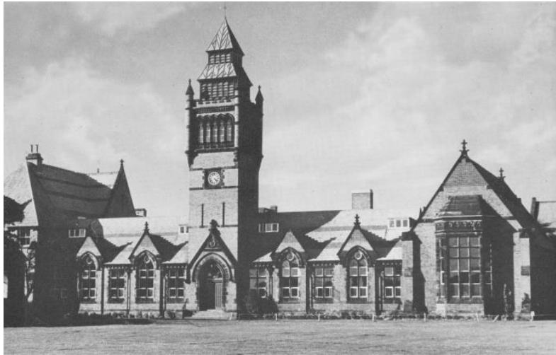
Main building of Merchant Taylors' School. This building, constructed in 1878, replaced the original main building constructed in 1620. The photo was taken in the late 1960s. (photo source Merchant Taylors' School)
