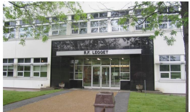
Left: Legget Avenue with R.F. Legget Building at the top of the photo (photo source Google Maps 2020). Above: Main entrance (photo by Harry Baker 2019)
