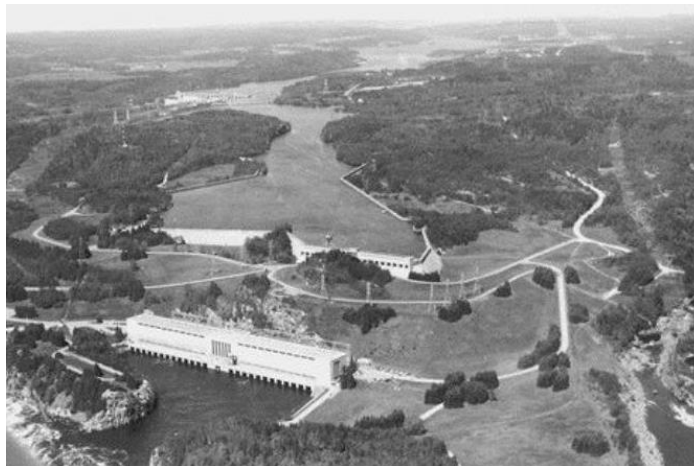
An oblique overview, looking upstream over the Shipshaw powerhouse (foreground) and Chute-à-Caron powerhouse (upper left). Date unknown. (photo source Northern Miner website)
