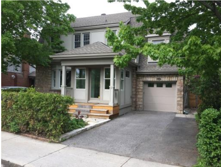
531 Echo Drive, Ottawa, Legget's home from 1947 to 1994 (Photo by Doug VanDine, 2019)
