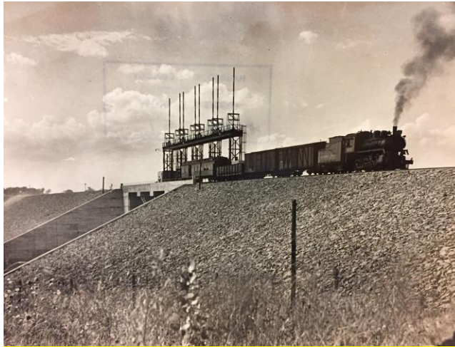
Fig 15.1 in Legget's and Paul Karrow's Handbook for Geology in Civil Engineering , published in 1983 by McGraw-Hill. The caption of this photo by Legget reads "The Shand Dam on the Grand River, Ontario, a dam built of glacial till with no core wall". Notice that Legget included a train in the photo.
