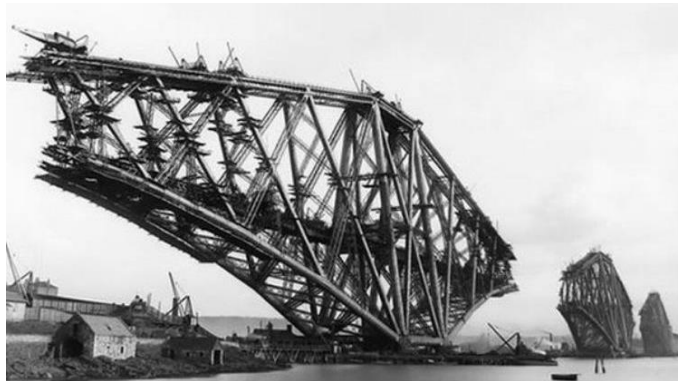
Firth of Forth Bridge under construction in the late 1880s (photo source BBC News website)
