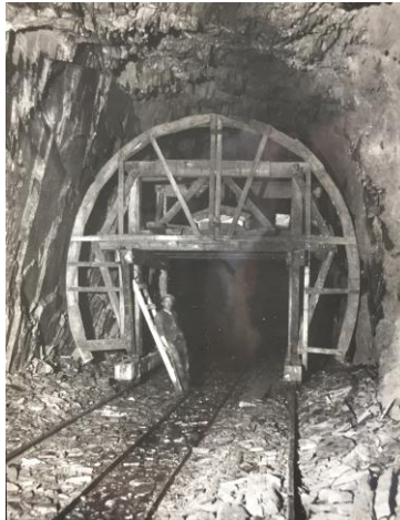
The Lochaber tunnel under construction (LAC Spec Coll)
