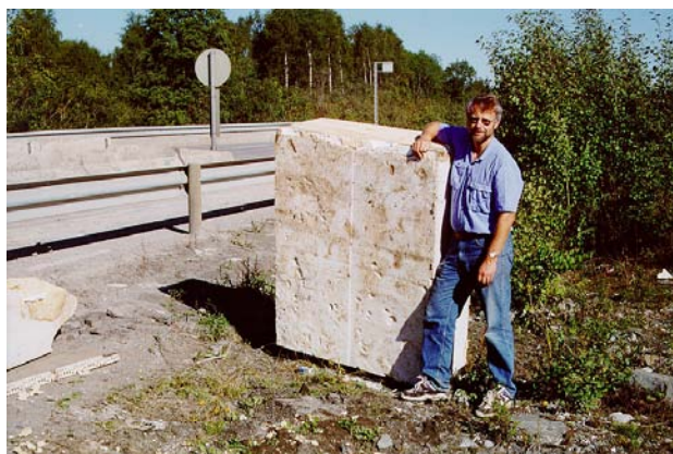
Figure 3. Excavation of a 24 years old EPS block from the first EPS embankment at Flom bridge
