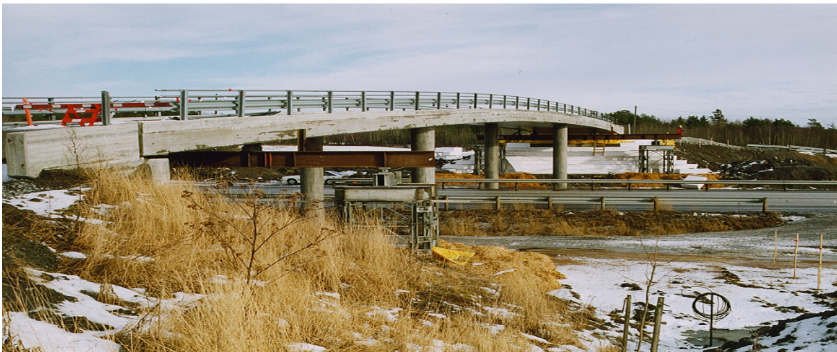
Figure 20. Temporary support of abutments at Hjelmungen
