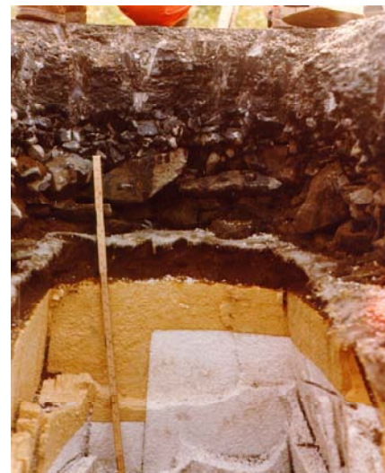
Figure 2. Excavation of the first EPS embankment at Flom bridge
