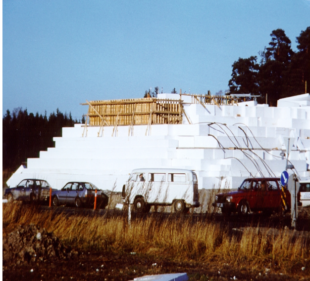
Figure 10. Construction of one abutment on the EPS embankments at Løkkeberg bridge.
