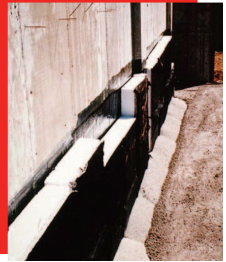
Graphic 8: Close-up of the geofoam product providing the functions of compressible inclusion, groundwater drainage, and thermal insulation in Kansas City [credit: GeoTech Systems Corporation].
