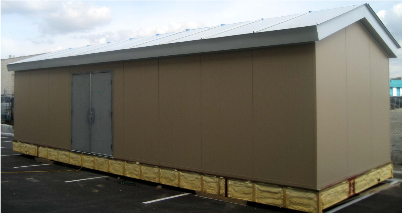
Energy efficient Structural Insulated Panels mounted on a 12 x 36 foot steel base.
