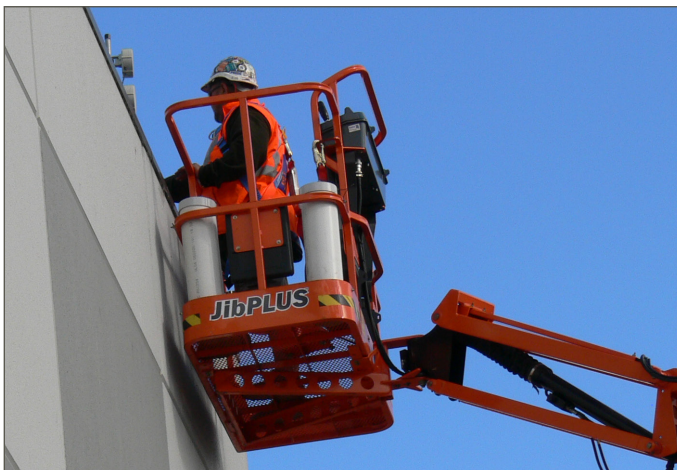
Figure 3. Minimal overhead structure in proximity
