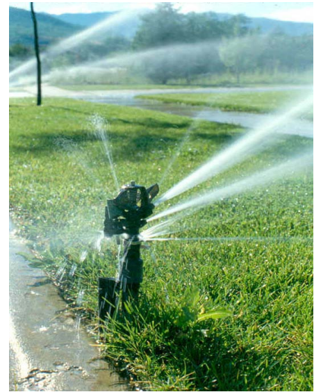
Watering at wrong time of day
