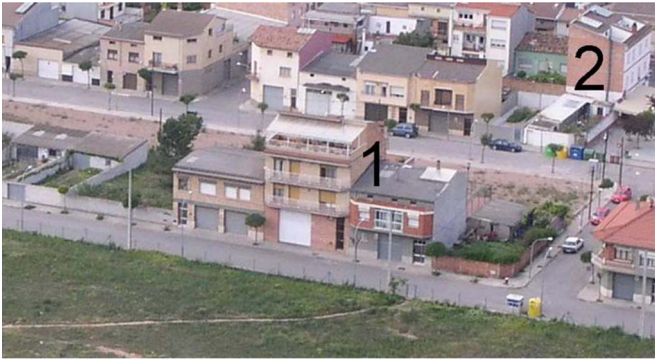
Fig. 2. Photograph of the neighborhood test site located in Sallent (50 km north from Barcelona, Spain) where subsidence monitoring with UPC's GB-SAR took place. Black numbers signal the structures modeled in Fig. 1.
