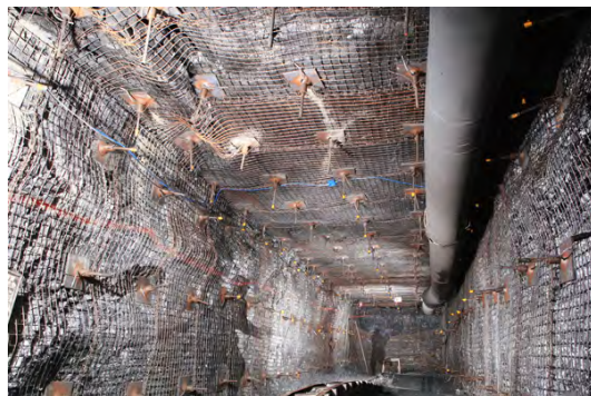
(a) Global photo of gas drainage gateway profile.
