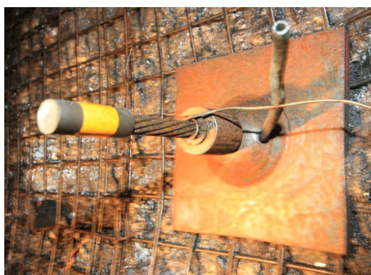
(b) Local photo of gas drainage gateway profile.
