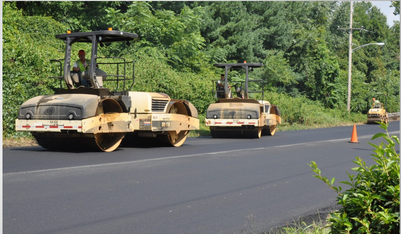
Compacting the First Pass
