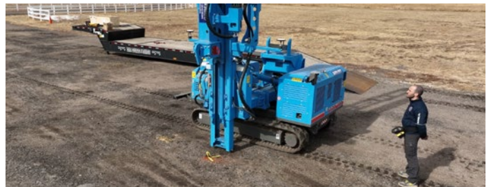
A FULLY AUTOMATED PILE DRIVER
