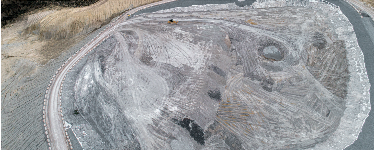
→ Cosentino®'s waste management plant
