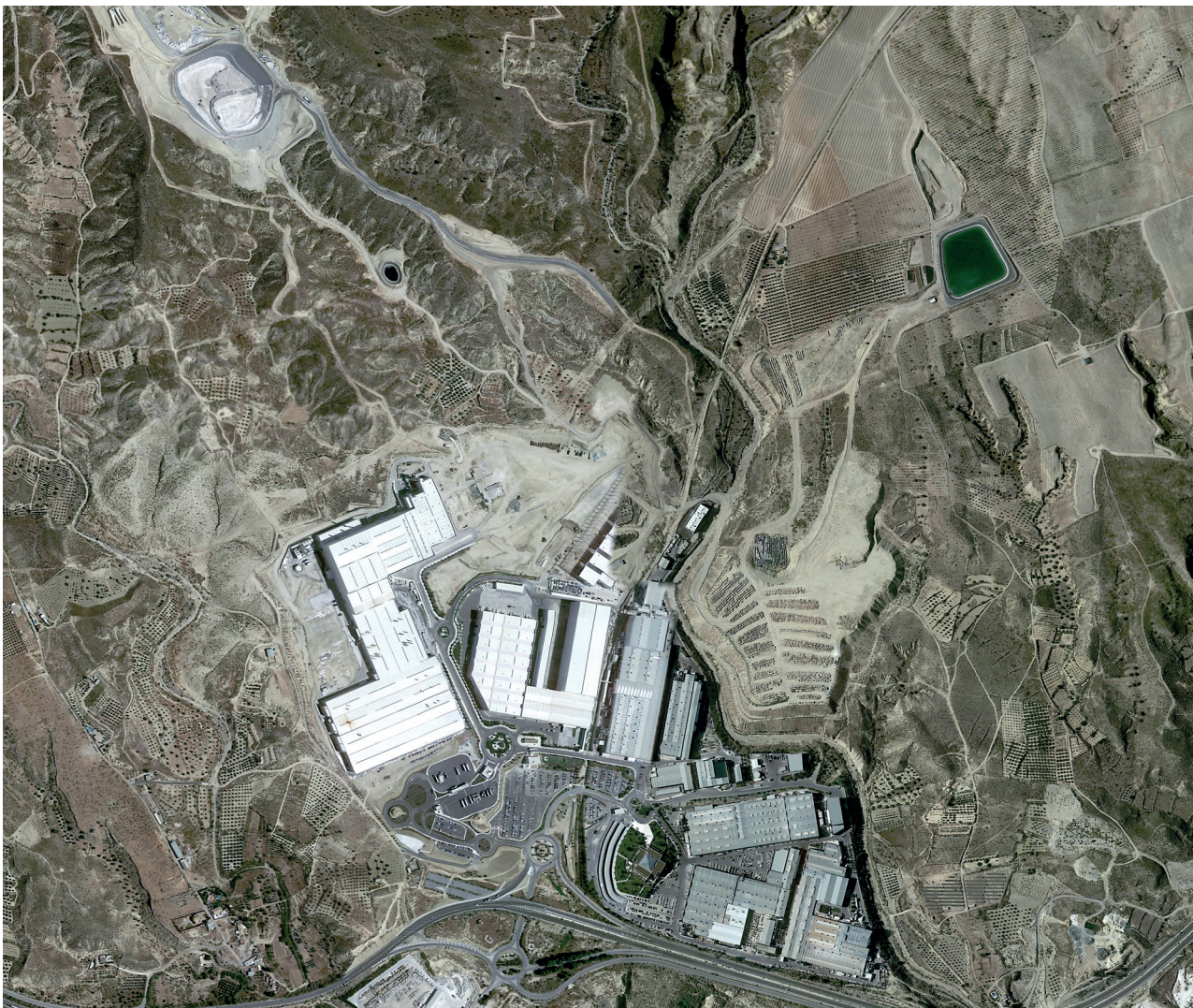
→ Aerial view of the Cosentino® industrial park
