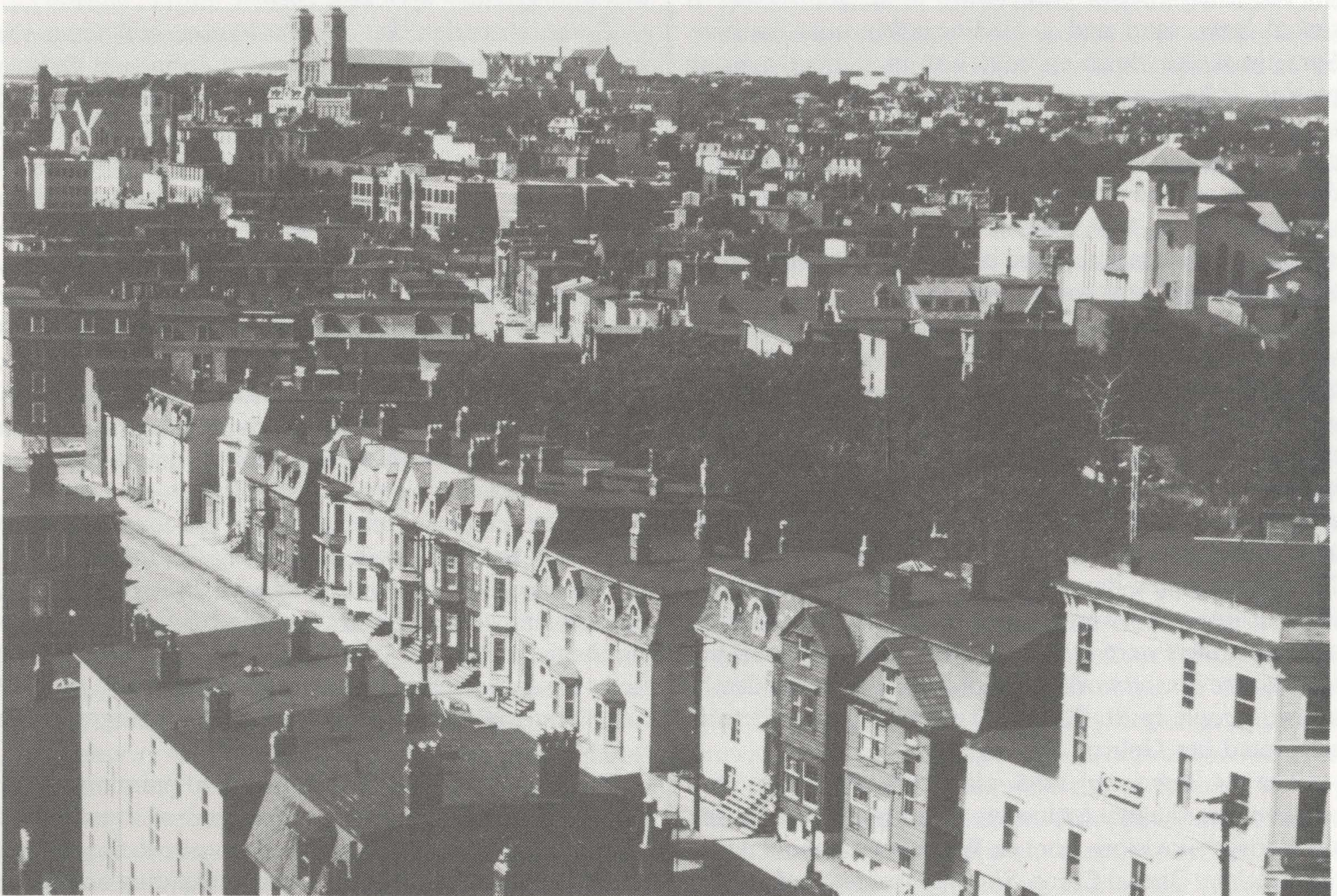
This row of elegant post-1892 houses on the north side of Gower Street still illustrates the profound influence of the Southcott's introduction of the Mansard roof to St. John's. While the fronts of some of these structures have been ruined by modern renovations the area is presently undergoing sensitive restoration.
