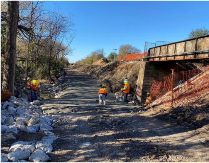
Placement of fresh concrete over rock berm in Dallas
