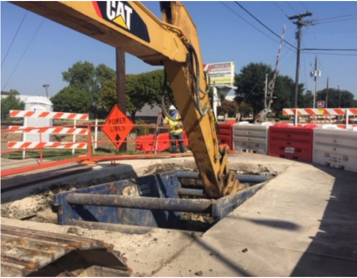
Excavating for a bore pit
