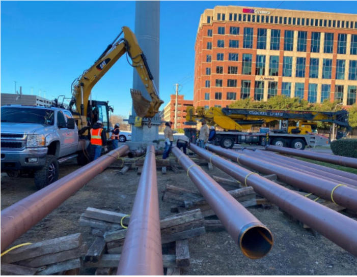
Welding pipe for Explorer pipeline at DNT and Knoll Trail
