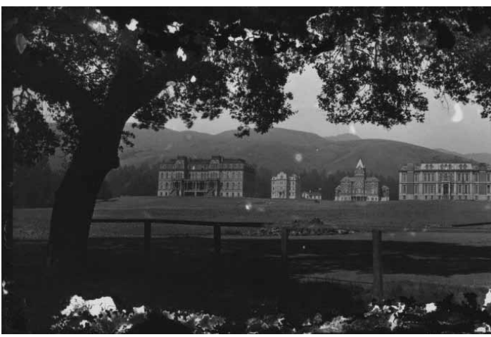
UC Berkeley, North and South Halls, 1900
