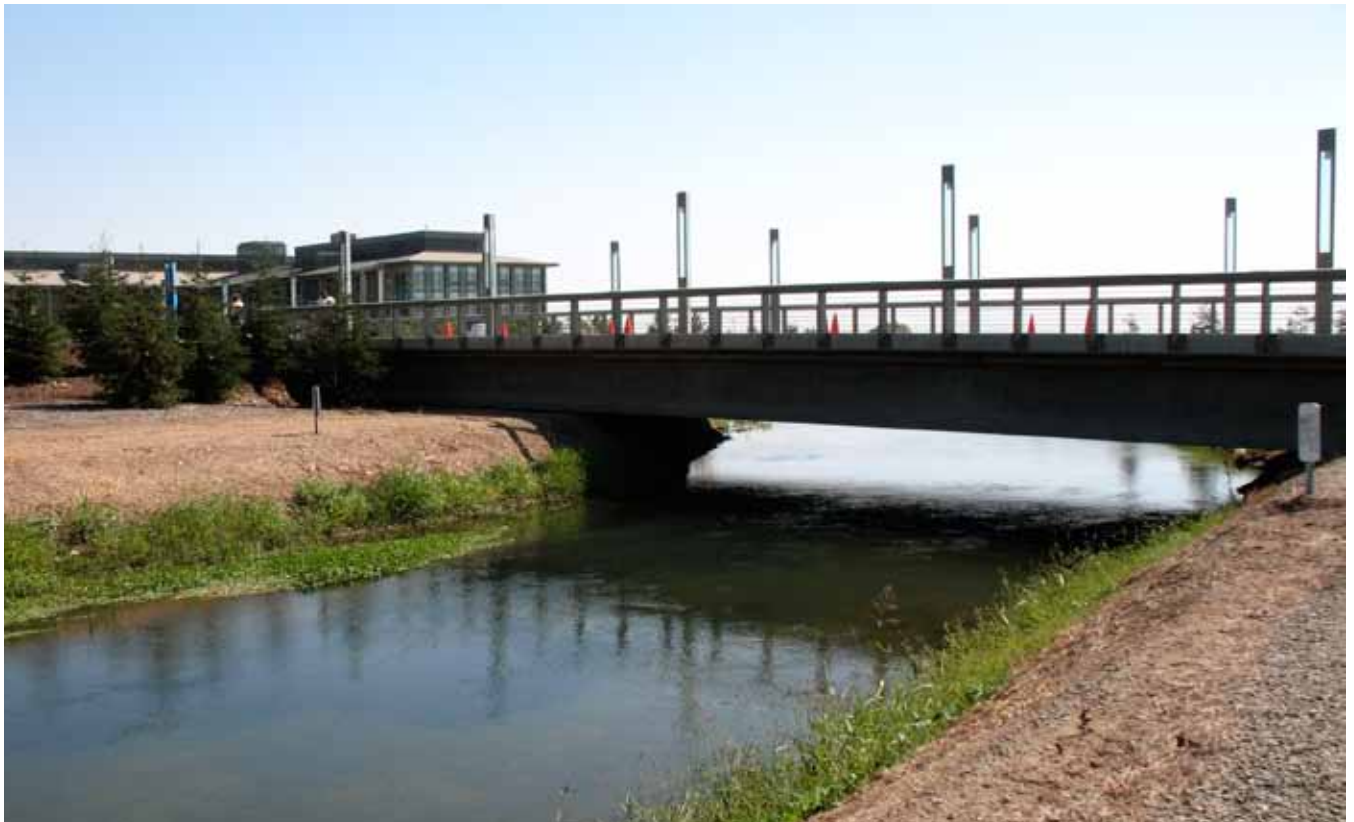
UC Merced's street and open space systems intersect with two agricultural irrigation canals owned by the Merced Irrigation District.
