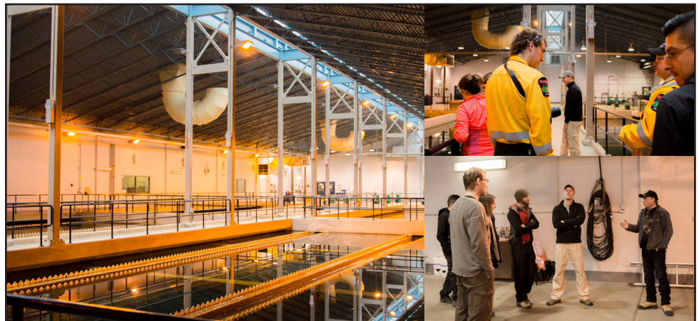
The group was treated to a tour of the Fort McMurray water treatment facility where they were taught about the work needed to keep the treatment plant up and running during the wildfire.
